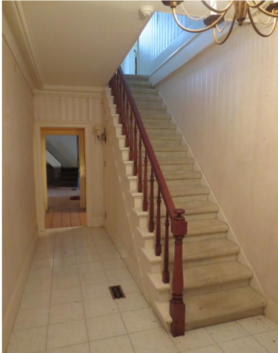
Front hall with stairway and plaster cavetto crown moulding
