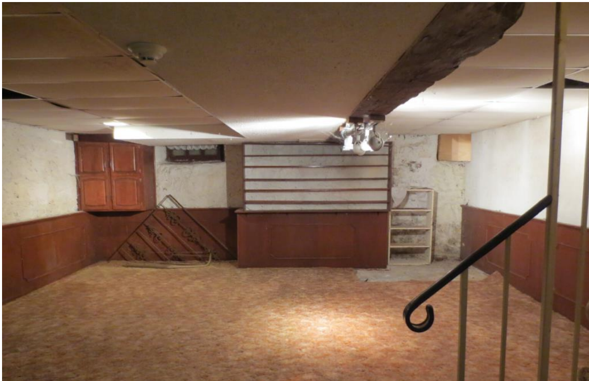
North room in basement with exposed heavy timber summer beam in ceiling
