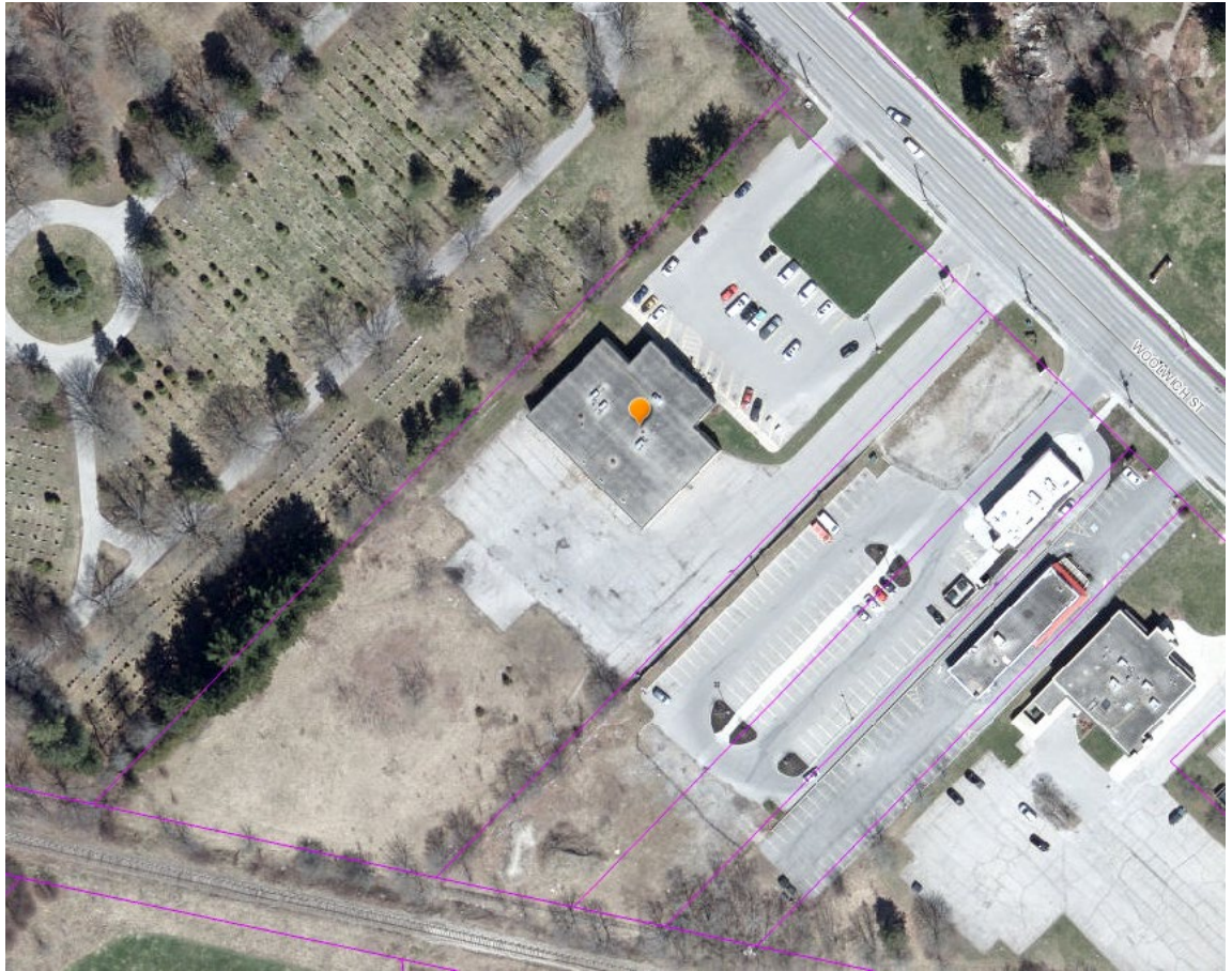
Figure 1: Aerial Image of the Subject Property (source GRCA Mapping)
