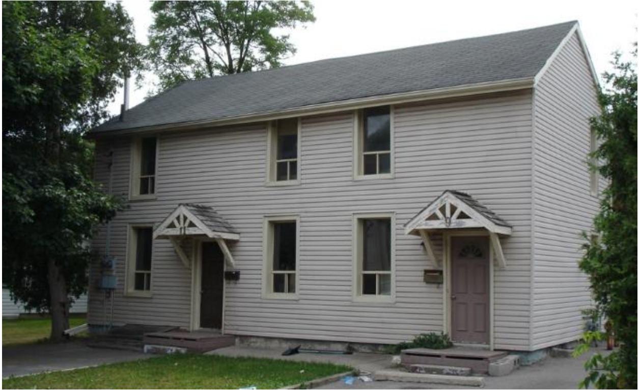
Figure 6 - 9 and 11 James St W in southeast corner of subject property (Photo: City of Guelph, 2005)
