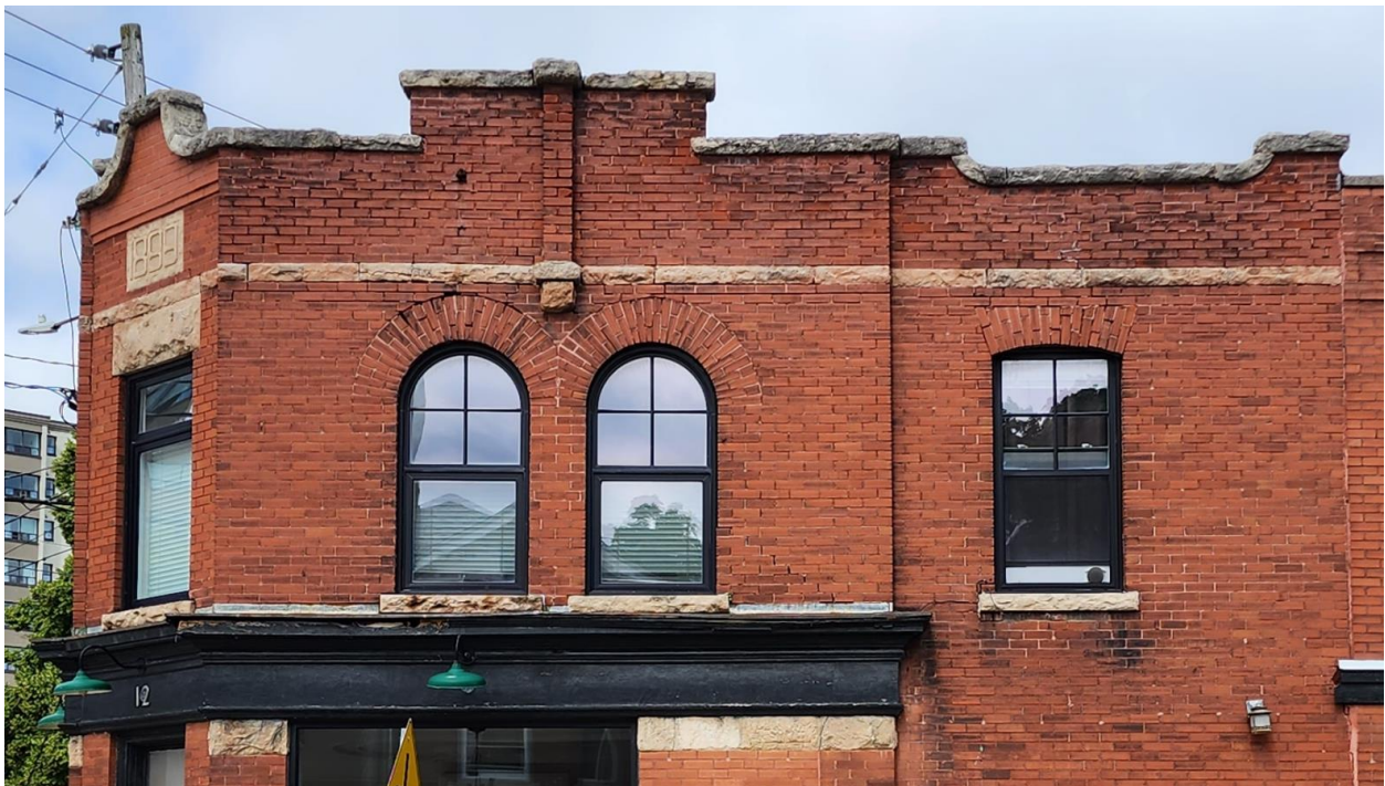
Figure 12: Coupled windows facing Eramosa Road. (Photo: S. Robinson, 2023)
