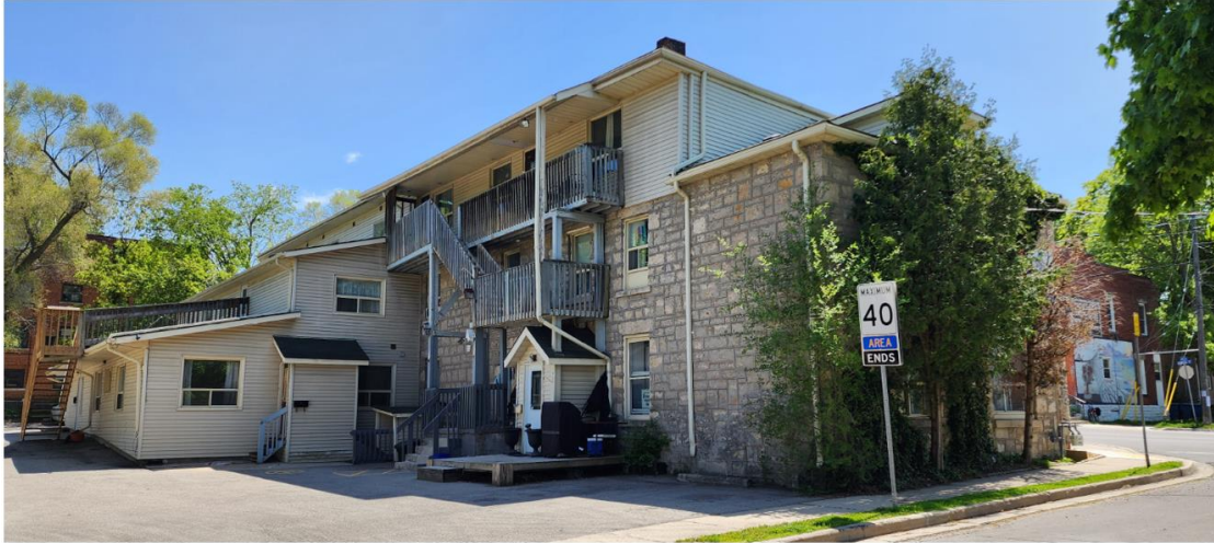
Figure 3 - 220 Gordon St, rear of the property viewed from north. (Photo: S. Robinson, 2023)
