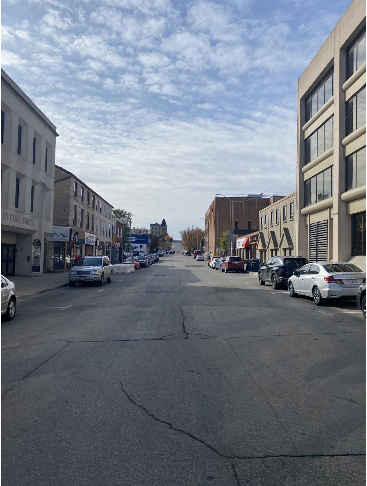
Figure 11: St Agnes viewed from the intersection of Cork Street and Wyndham Street
