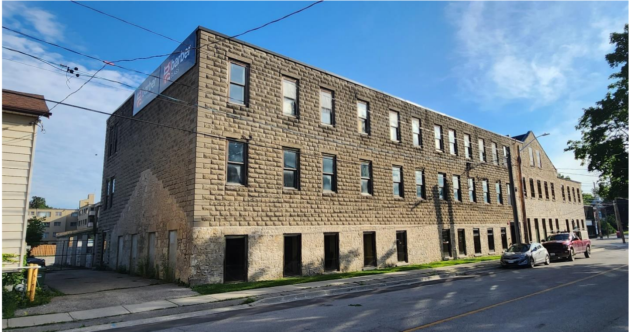
Figure 3 - Image of 167 Suffolk Street West, facing north (S. Robinson 2023).
