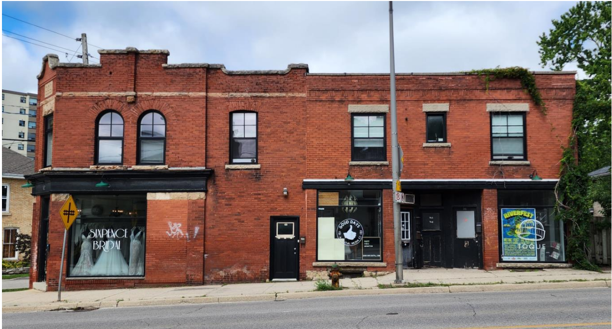
Figure 13: Eramosa Road elevation. (Photo: Sr. Robinson, 2023)
