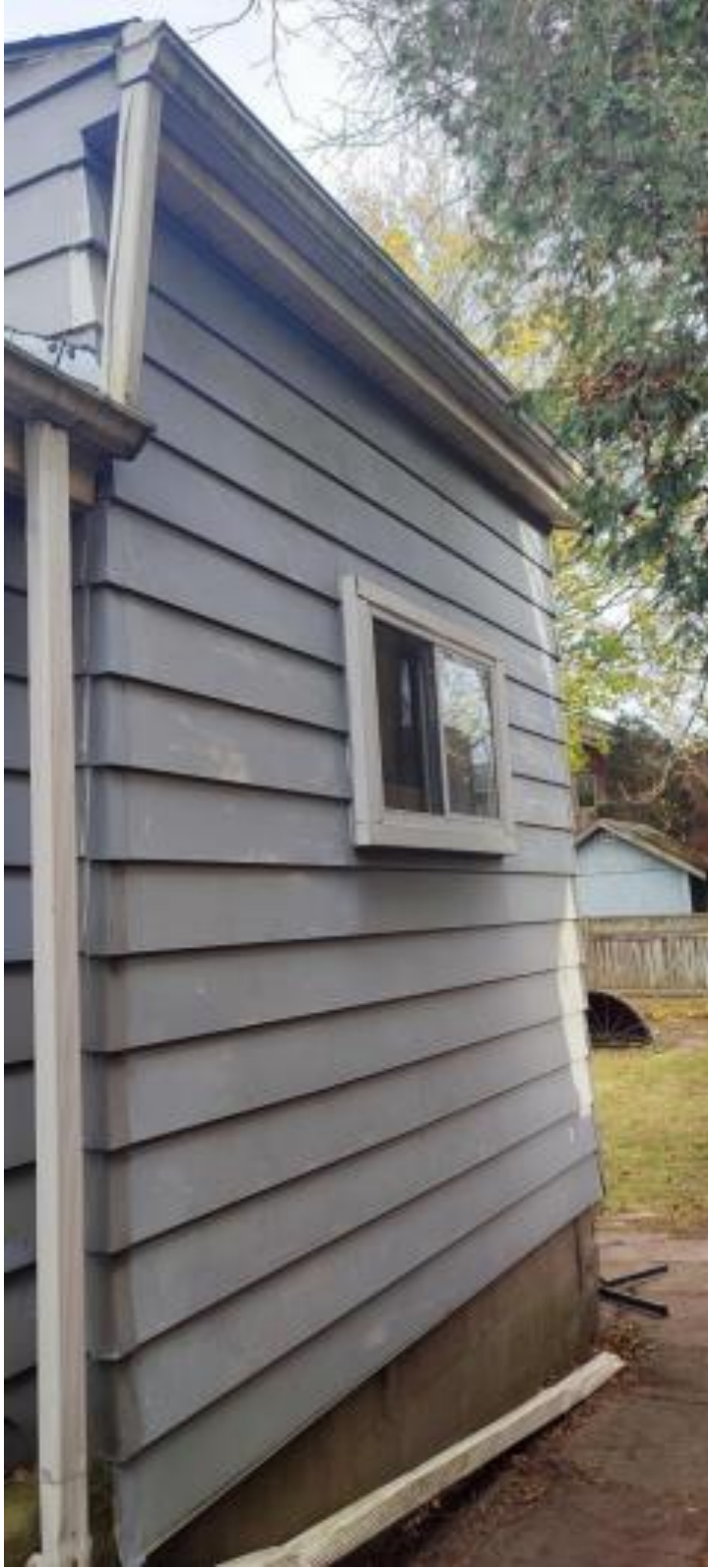
Figure 4: West elevation of the 1967 addition
