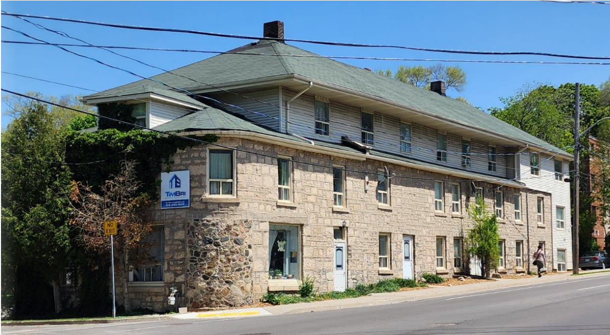
Figure 2 - 220 Gordon St, View from the south, 220 Gordon St (Photo: S. Robinson, 2023)
