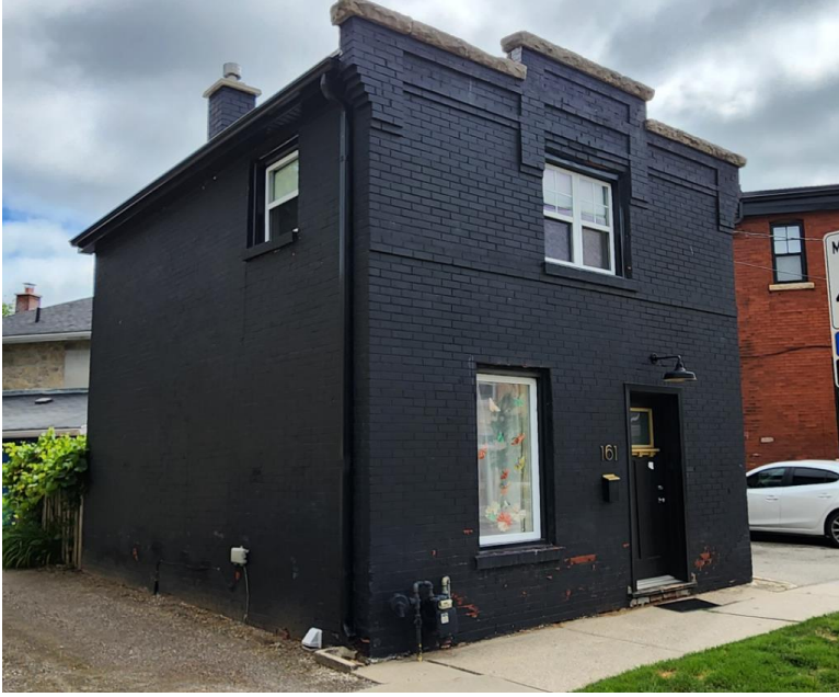
Figure 16: View of stable building from west. (Photo: S. Robinson, 2023)
