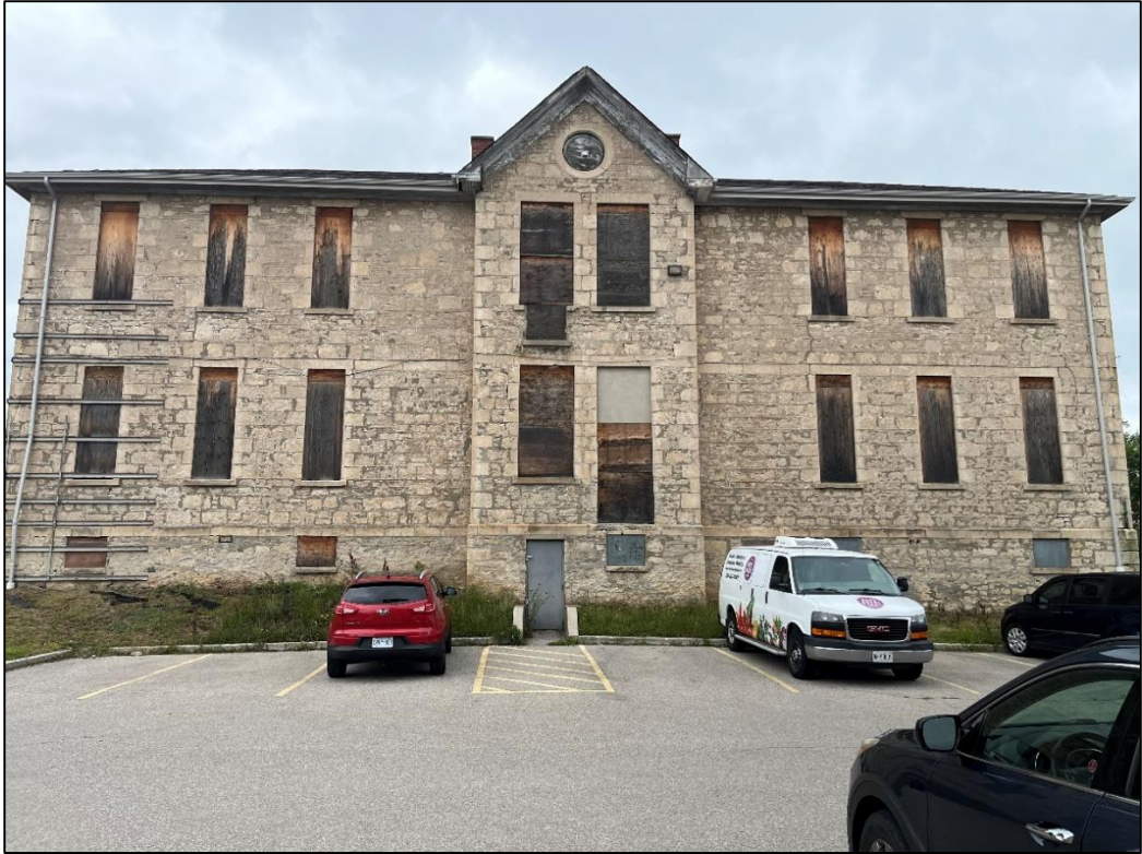
Figure 6: Southern (rear) façade of the building
