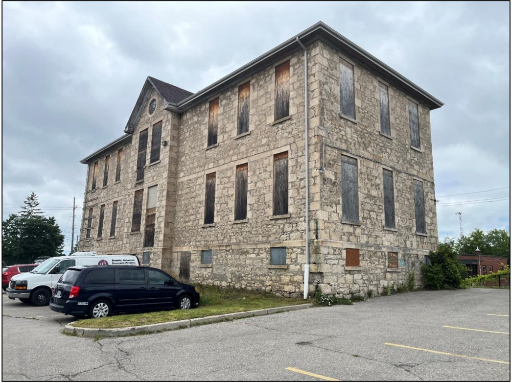
Figure 7: Southeast corner of the building
