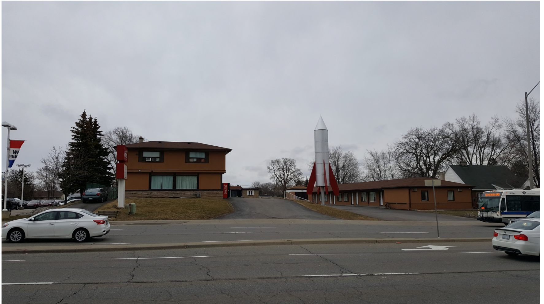
View of site looking east from Hespeler Road.
