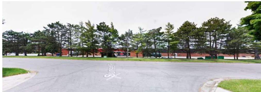
4 View of the site facing south from intersection of Sunset Rd and Applewood Crescent
