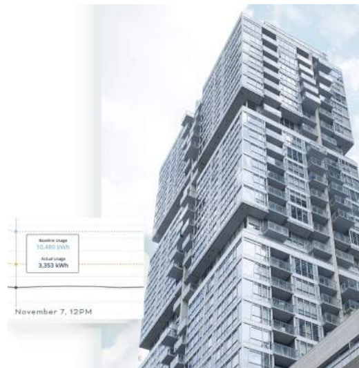
Building Automation Systems achieve up to 30% lower consumption of electricity and gas
