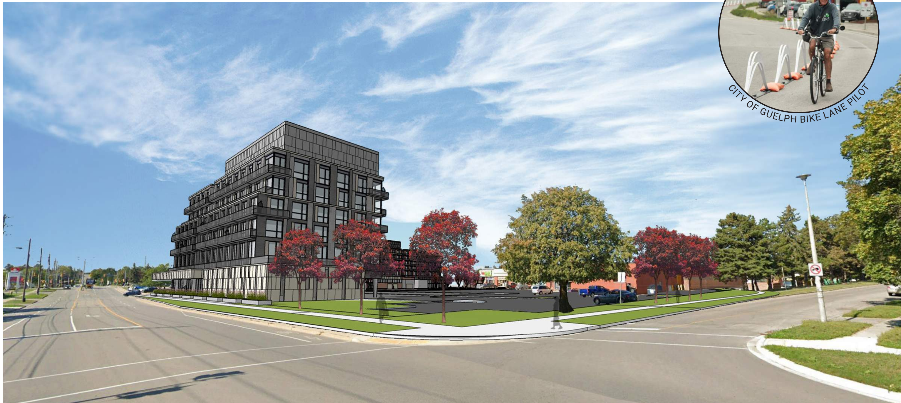
Building G - View from Willow Rd and Applewood Crescent
