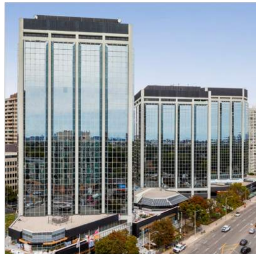
Artificial Intelligence based system to manage energy resources to reduce peak power consumption
