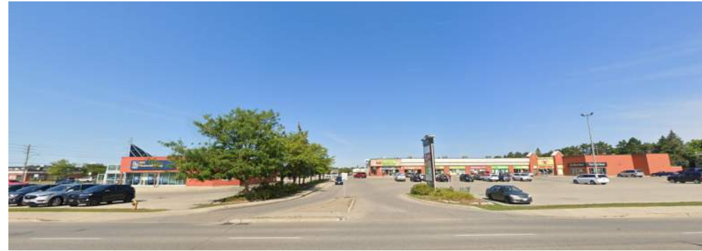
2 View of the site facing west from Willow Rd at midblock access point
