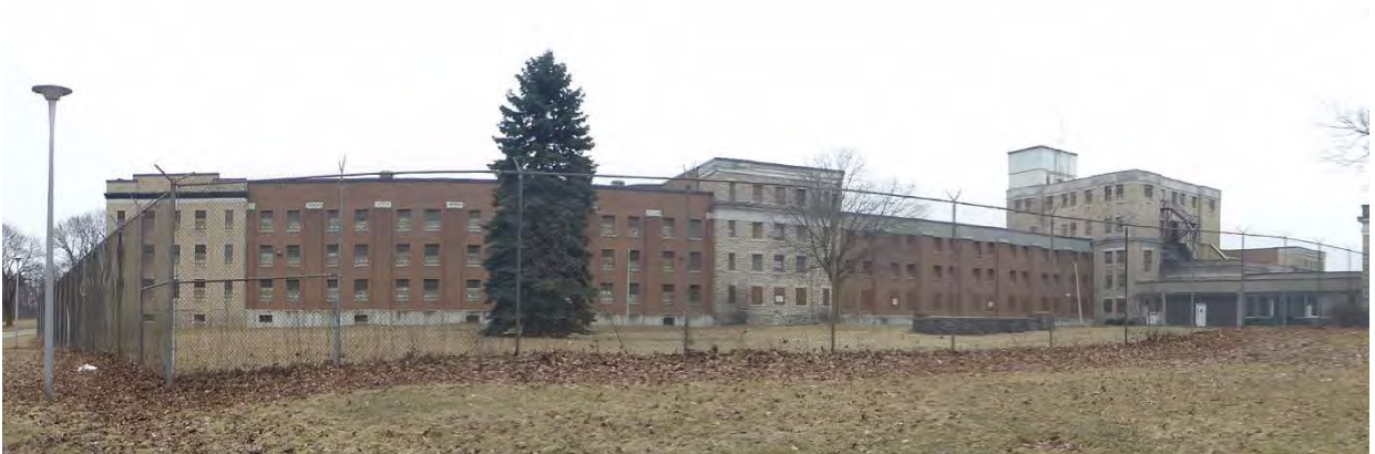
North Elevation of C Cells (B13434) and Tower & Main Corridor (B13431)
