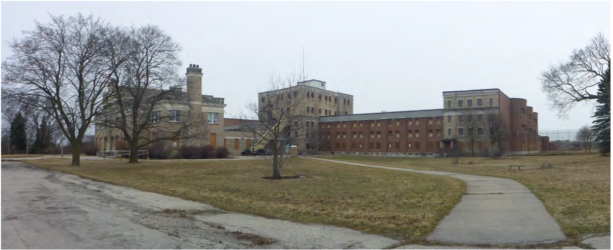
GCC from parking lot (looking South-East)
