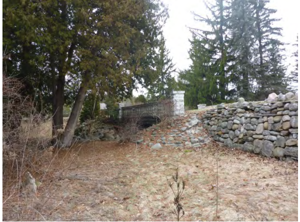
Stone wall and stone bridge
