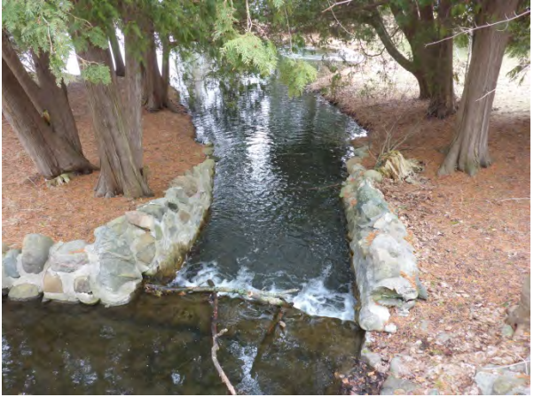
Stone wall lined watercourse
