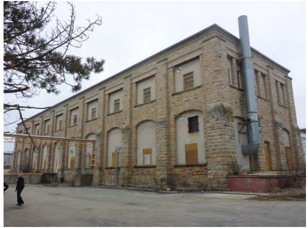
Machine Shop (B13450) – West Elevation
