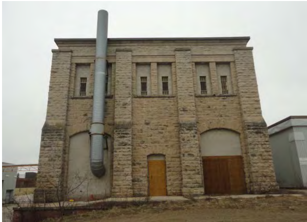
Machine Shop (B13450) – South Elevation
