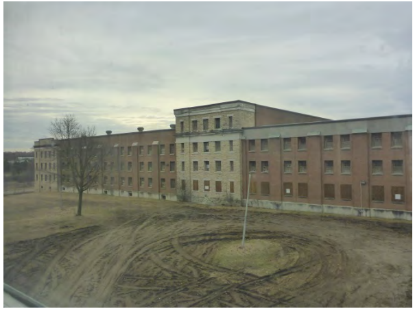
North Elevation of C Cells (B13434)
