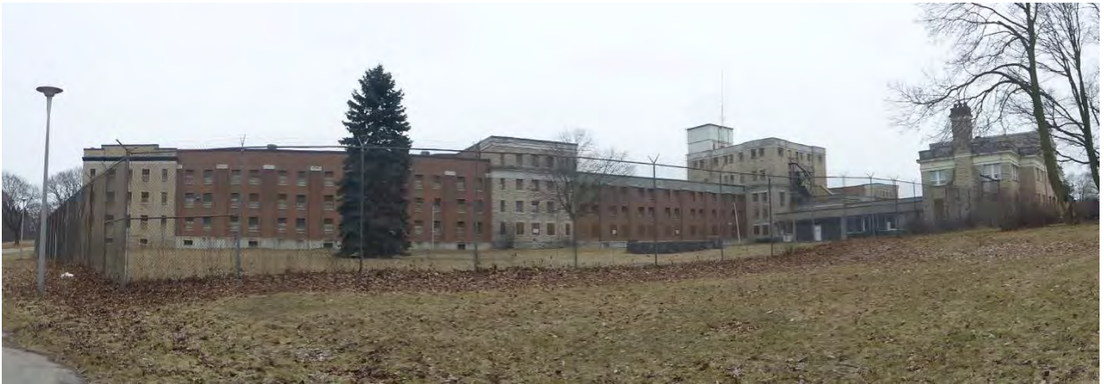
GCC from driveway (looking South-West)
