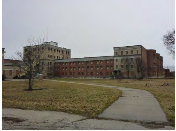
North Elevation of B Cells (B13432) and Tower & Main Corridor (B13431)
