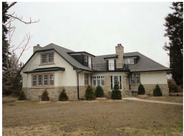
Superintendent's Residence (B13499) - West Elevation
