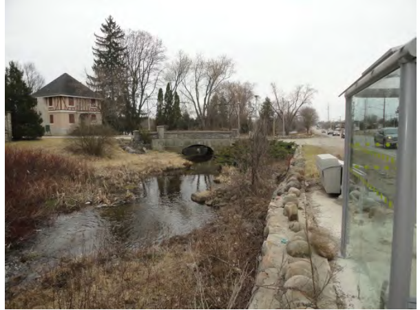
Willowbank Hall, stone bridge, stone wall along York Road
