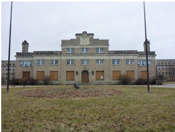
North Elevation of Administration Building (B13430)
