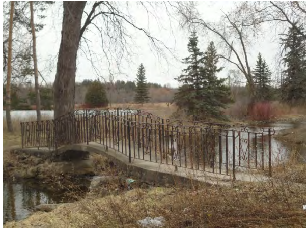
Bridge crossing watercourse along York Road
