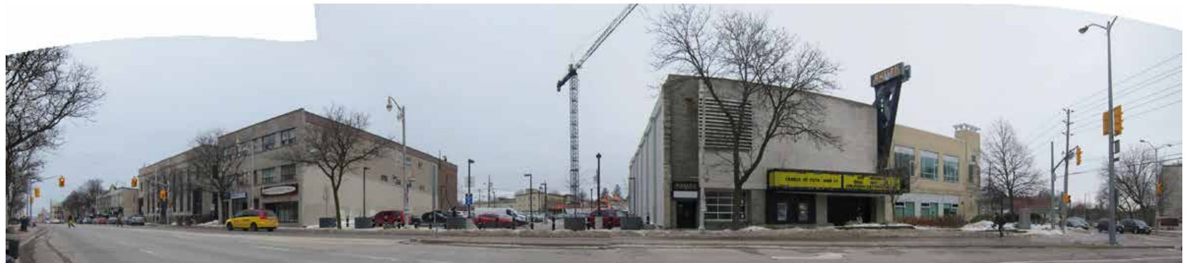
Figure 18 Panorama of Wyndham Street looking west with 146 and 166 Wyndham Street North properties visible in the foreground
