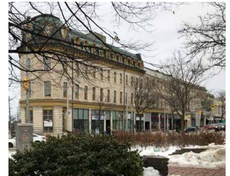
Figure 49 Wyndham Street North buildings representative of the rich limestone materiality of downtown Guelph
