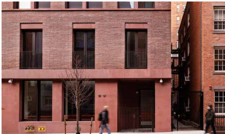
Figure 63 Material Precedent - brick texture and complementary flat panel
