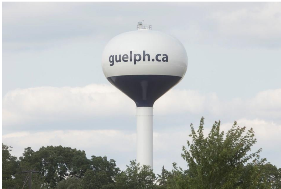
Figure 2 Speedvale Water Tower (example of elevated water storage)
