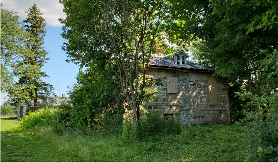
Farmhouse and shed from driveway
