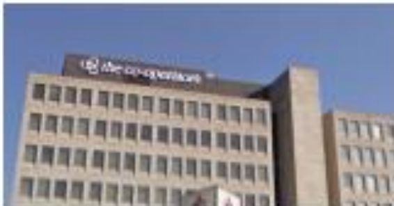
Co-Operators – MacDonnell Street (South elevation)
