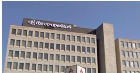
Co-Operators – MacDonnell Street (South elevation)
