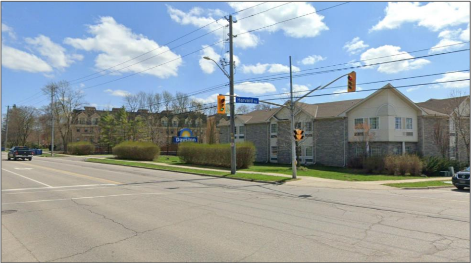
View of the Site from Gordon Street (East)
