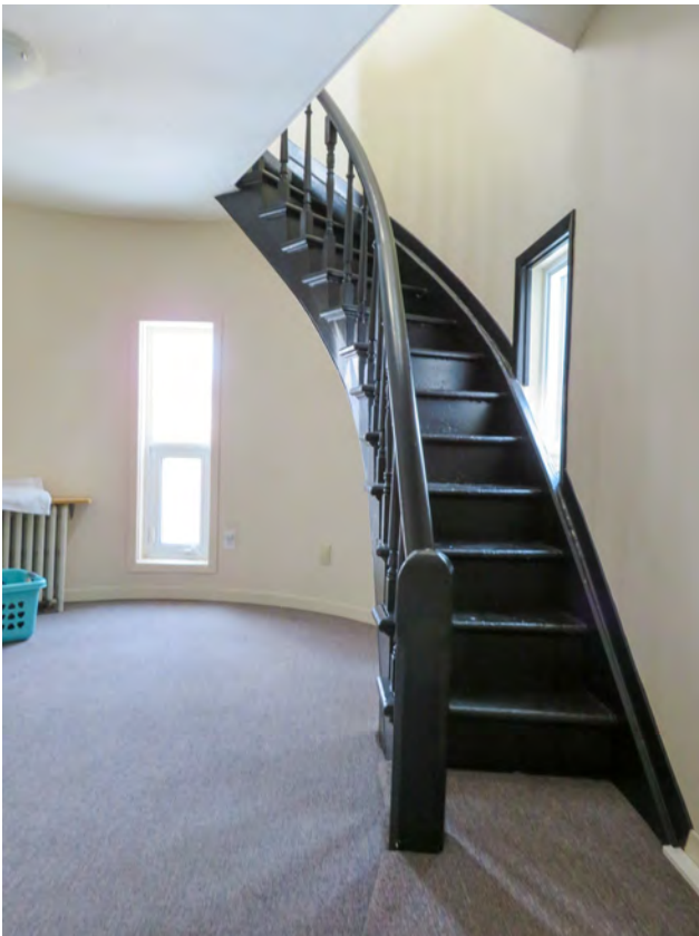
c.1860 STAIRCASE – CURVED WOOD STAIRCASE AT THE TOP OF THE TOWER [UNIT R2B]
