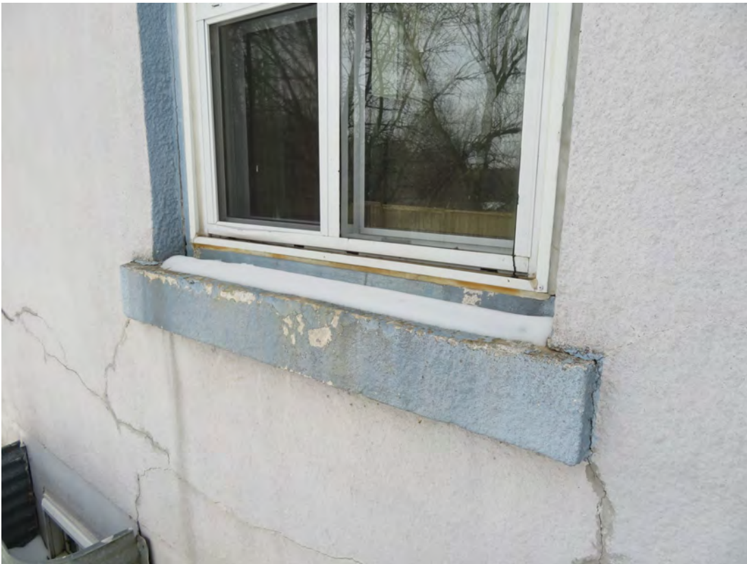
EAST ELEVATION – WINDOW SILL
