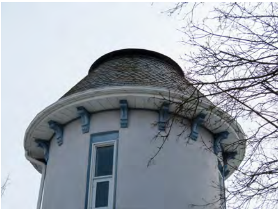
TOWER ON THE NORTH ELEVATION
