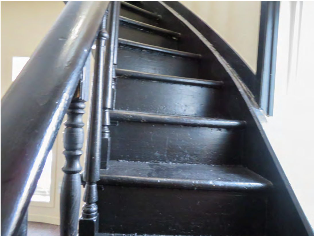
c.1860 STAIRCASE – CURVED WOOD STAIRCASE AT THE TOP OF THE TOWER [UNIT R2B]
