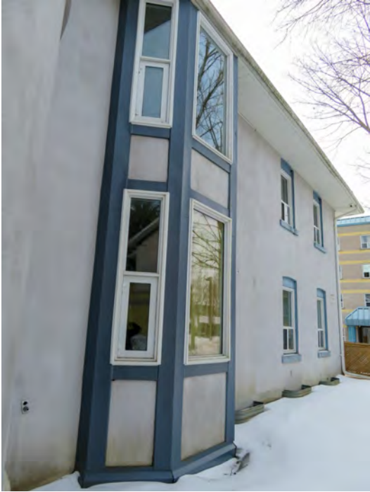
NORTH ELEVATION – WINDOWS
