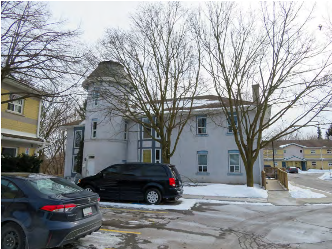
2022 PHOTO - converted to apartments – vinyl windows installed and bay window added – cement stucco extended down to grade
