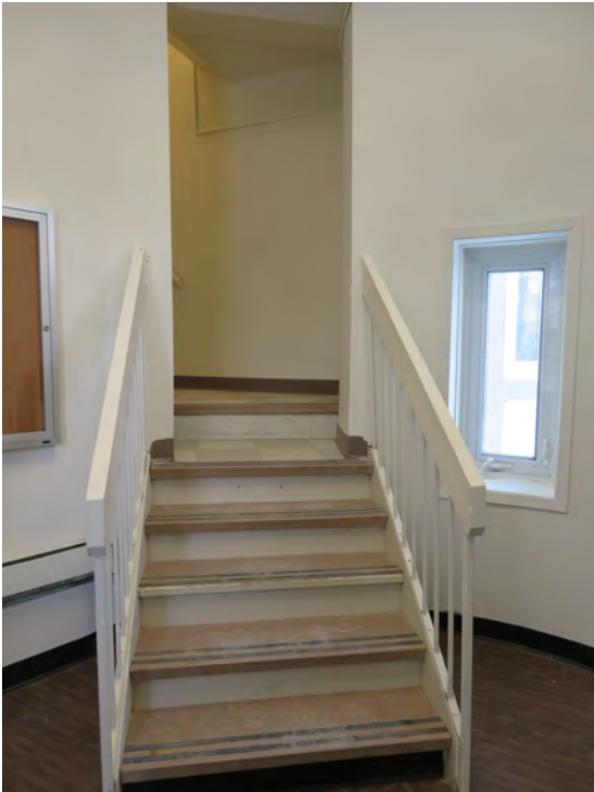
NORTH STAIRWELL AT THE BASE OF THE TOWER
