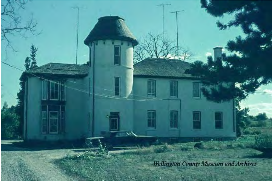
1973 PHOTO - masonry coated with paint or stucco [Wellington County Museum & Archives]
