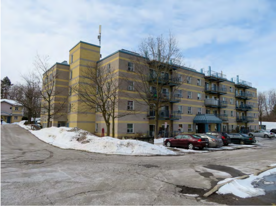
VIEW LOOKING WEST TOWARDS THE APARTMENT BUILDING ON THE SUBJECT PROPERTY
