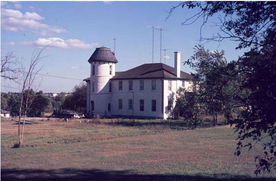
1973 PHOTO - masonry coated with paint or stucco
