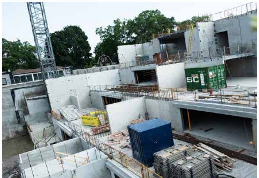
The photo to the right shows 3 stories of underground parking being constructed at 71 Wyndham South.
