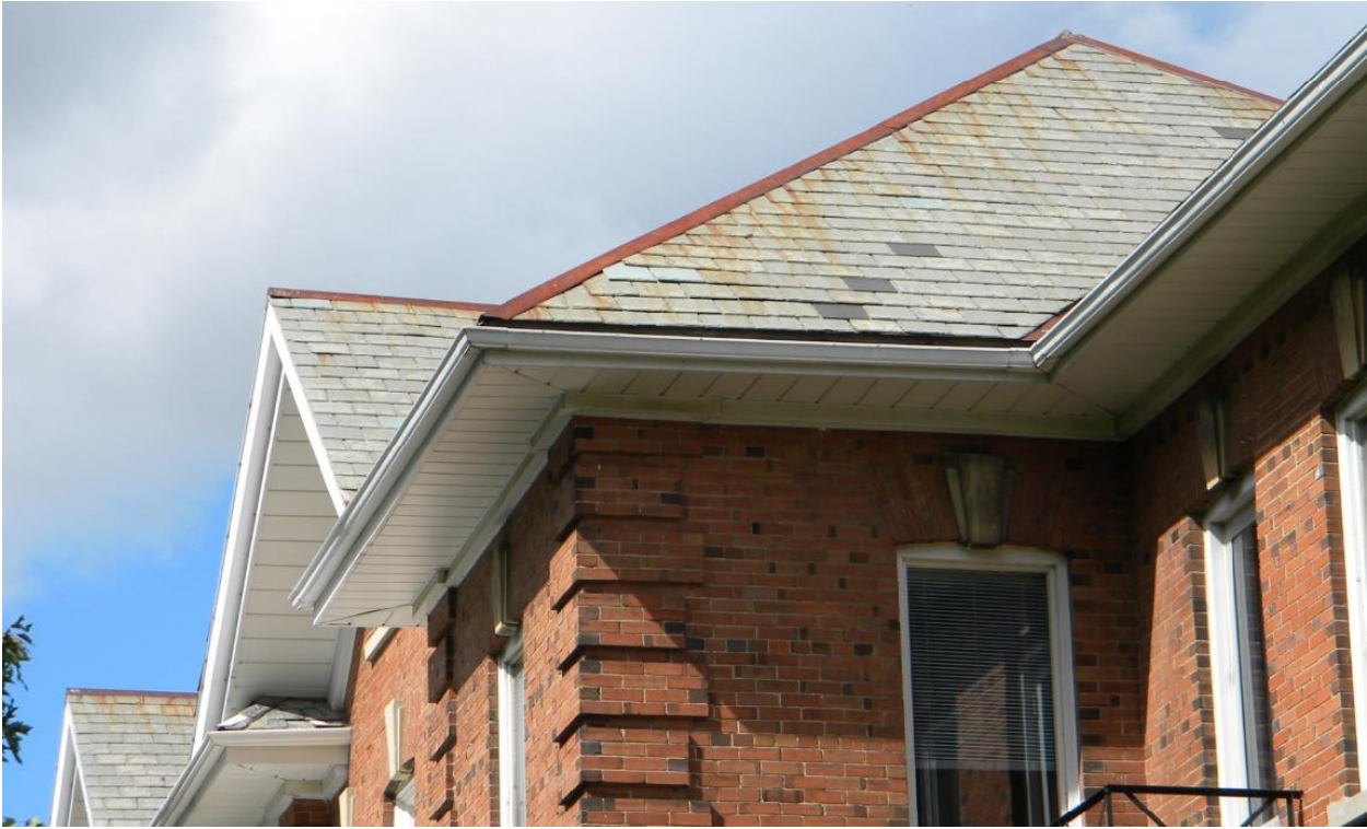
Figure 23 - Slate roof (Photo 2012)
