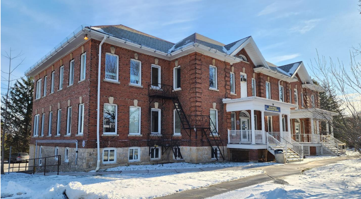
Figure 18 - 65 Delhi Street (view from west) (Photo 2022)
