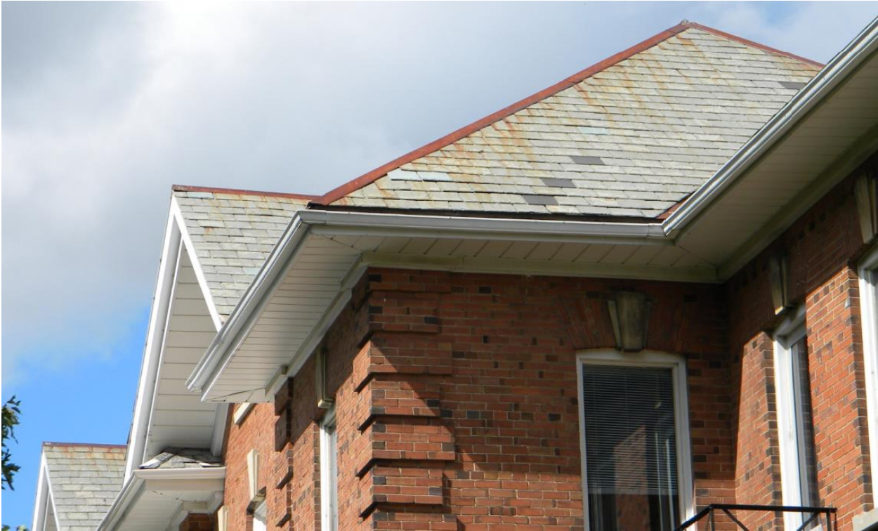
Figure 23 - Slate roof (Photo 2012)
