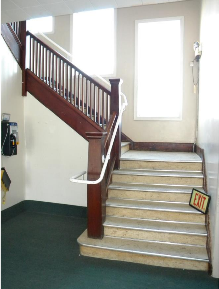
Figure 26 - Interior stairway (Photo 2013)
