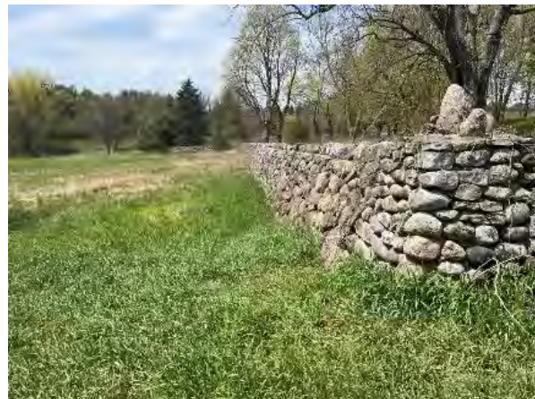
Image 85: Fieldstone retaining wall
