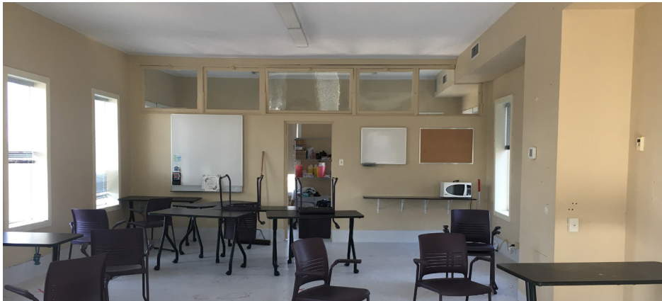
View of the infirmary space in the east wing top floor, with plaster walls and ceiling. Mechanical systems have been added and covered with gypsum board on the right vertical shaft and bulkhead vents at the ceiling.
