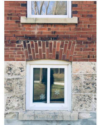
View of 'squared stonework' with ribbon mortar joint. Cracked stone sills of both windows show the path of water and deterioration.
