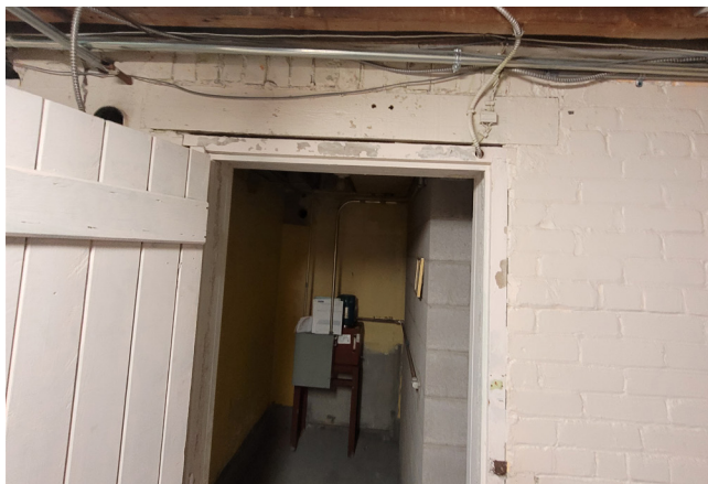
View into the elevator room with the concrete block elevator shaft on the right. The elevator capacity is for 2 people according to the posted certificate, and not in compliance with current accessibility codes.
