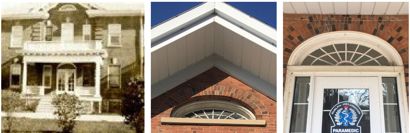
Images showing remaining original wood windows as seen in the c. 1941 photo left, and current views today: the semi-elliptical gable window and the arched window transom above the door. Both will be maintained as part of the annual maintenance program.
