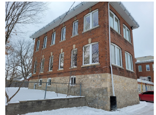
View of the south-west building corner showing the projecting brick coursing with blackened top edge becoming prominent.
