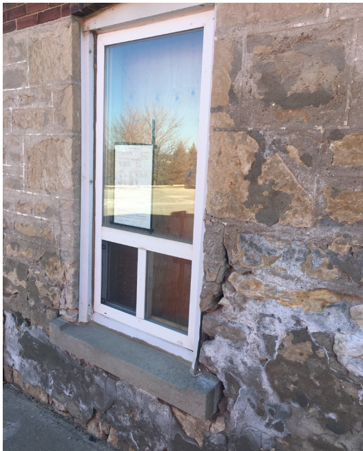
Image showing build up of efflorescence (white area) on the stone caused by use of impermeable mortars which should be removed and repointed with lime-based mortar.
