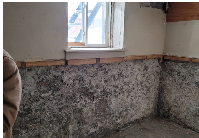
View of north wall section with fire escape visible outside the window. The north wall has been heavily parged likely intended to stop moisture on the surfaces below grade.
