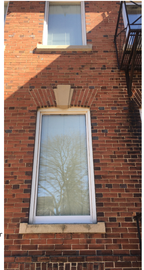
View showing original limebased mortar on the brick wall with repairs and cracked joints below the lower window sill.
