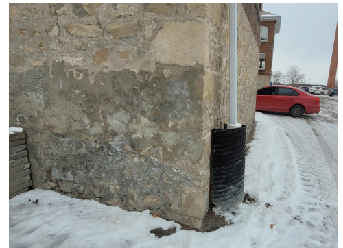
Stone foundation wall repair at the south-east building corner. Cement-based mortar causes water to migrate to more permeable areas and vulnerable to freeze/thaw
