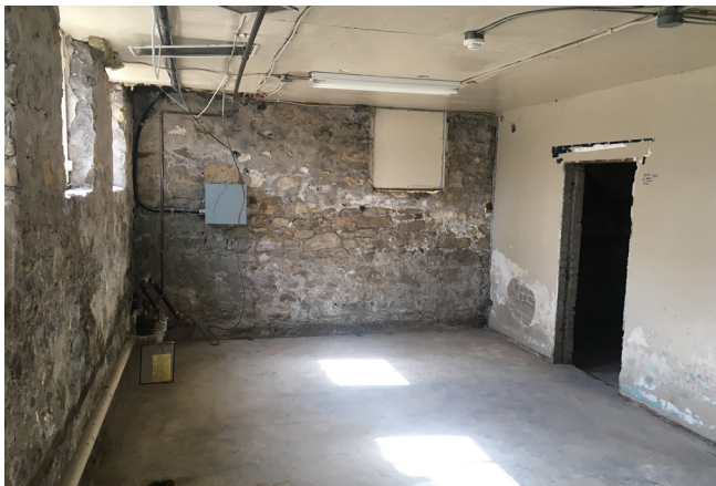
View of north-east wall (end) with mortar covering the stone on the left corner and across the wall top and bottom. The white sloped band indicates efflorescence where water has leached minerals from the stone and mortar work along the line between subgrade and above grade conditions.
