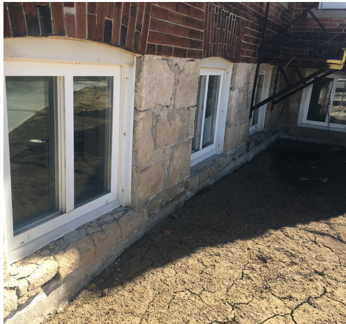
Image showing example of deteriorating masonry conditions. Foundation walls should be repointed with lime-based mortar and the broken stone sills replaced to protect the building from water infiltration.
