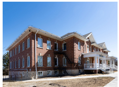
View of the south-west corner of the building showing replacement vertical sliding windows at the foundations.
