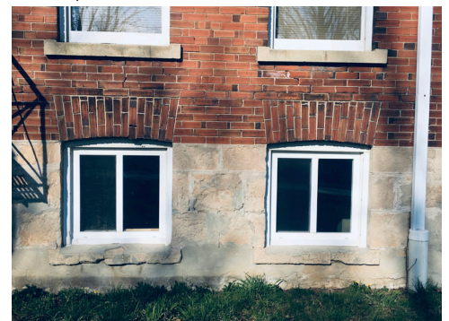
Stone foundation wall repairs and missing stone lintel sections on the lower windows.
