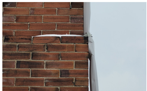
Detail view of the projecting brick coursing with deteriorated and missing mortar below the snow accumulation.
