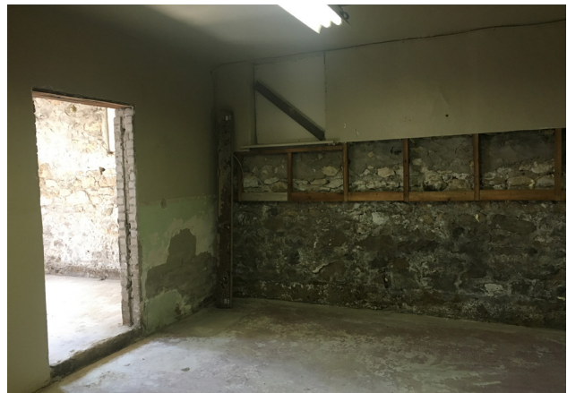
View of east wall section with mortar repair behind the added partial furring with insulation of the top section. Load-bearing brick masonry wall on the left shows some failing plaster but is otherwise in solid condition.
