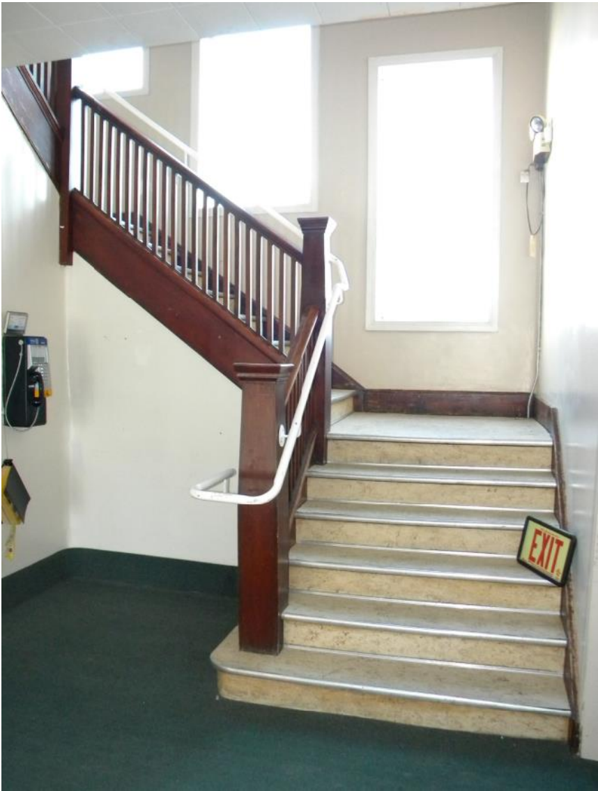
Figure 9 - Interior stairway (Photo 2013)
