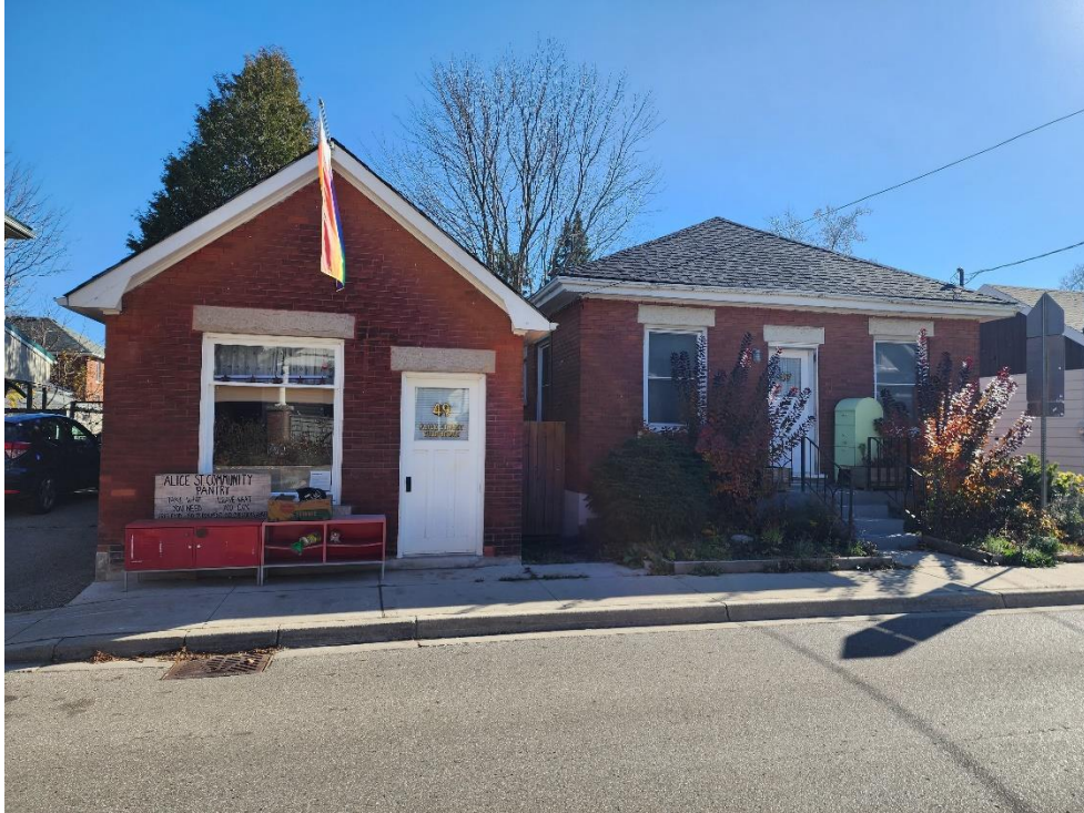
Figure 2 – 47 Alice Street (facing south) (Photo 2022 – S. Robinson)
