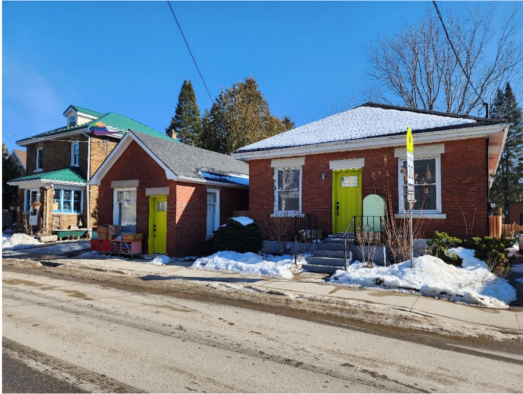
Figure 1 – 47 Alice Street (facing south) (Photo 2023 – S. Robinson)
