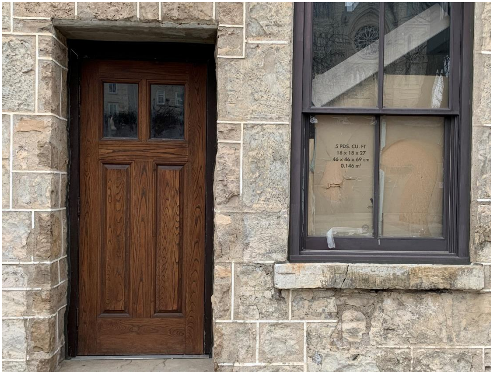
Figure 4 – 49 Norfolk St, entrance off Norfolk Street, left of main entrance (facing northeast) (Photo 2023 – V. Nagy)
