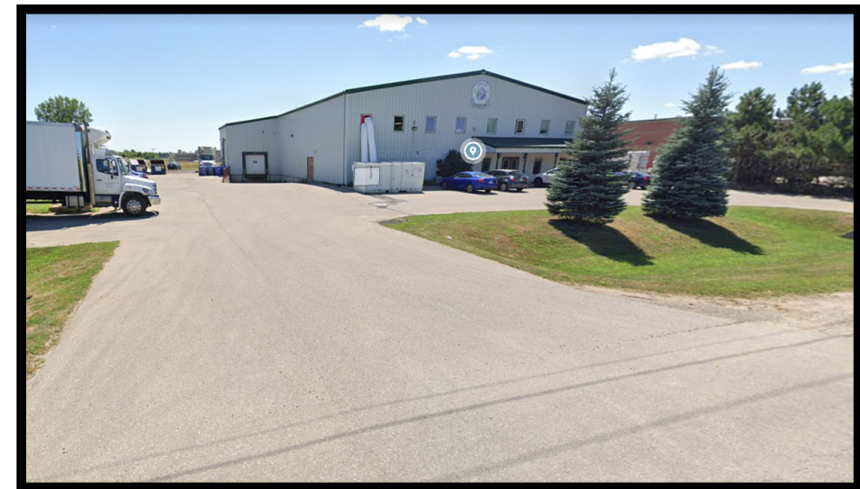
FIGURE #4 EXAMPLE OF LOADING DOCK DOOR AND RETAINING WALL LOCATED ON FRONT OF BUILDING FACING FRONT STREET.
