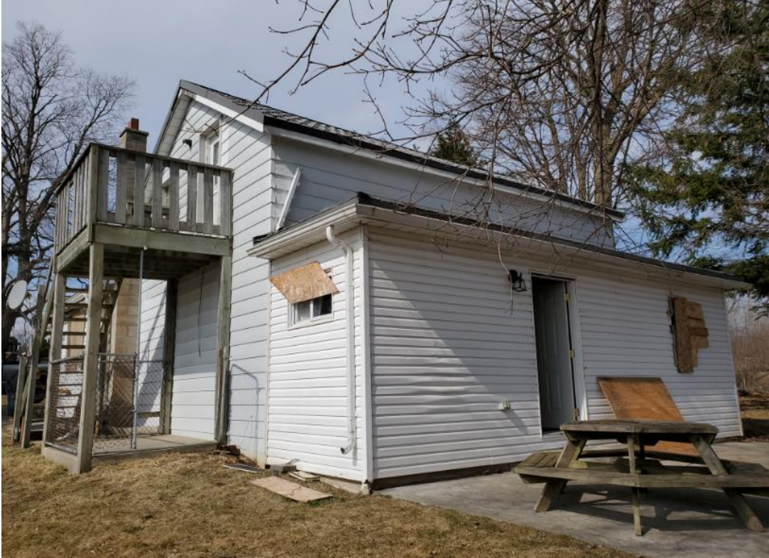
Figures 5 and 6 - Dwelling seen from south and north
