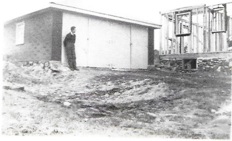
Gerdie standing at the garage watching building in progress.
