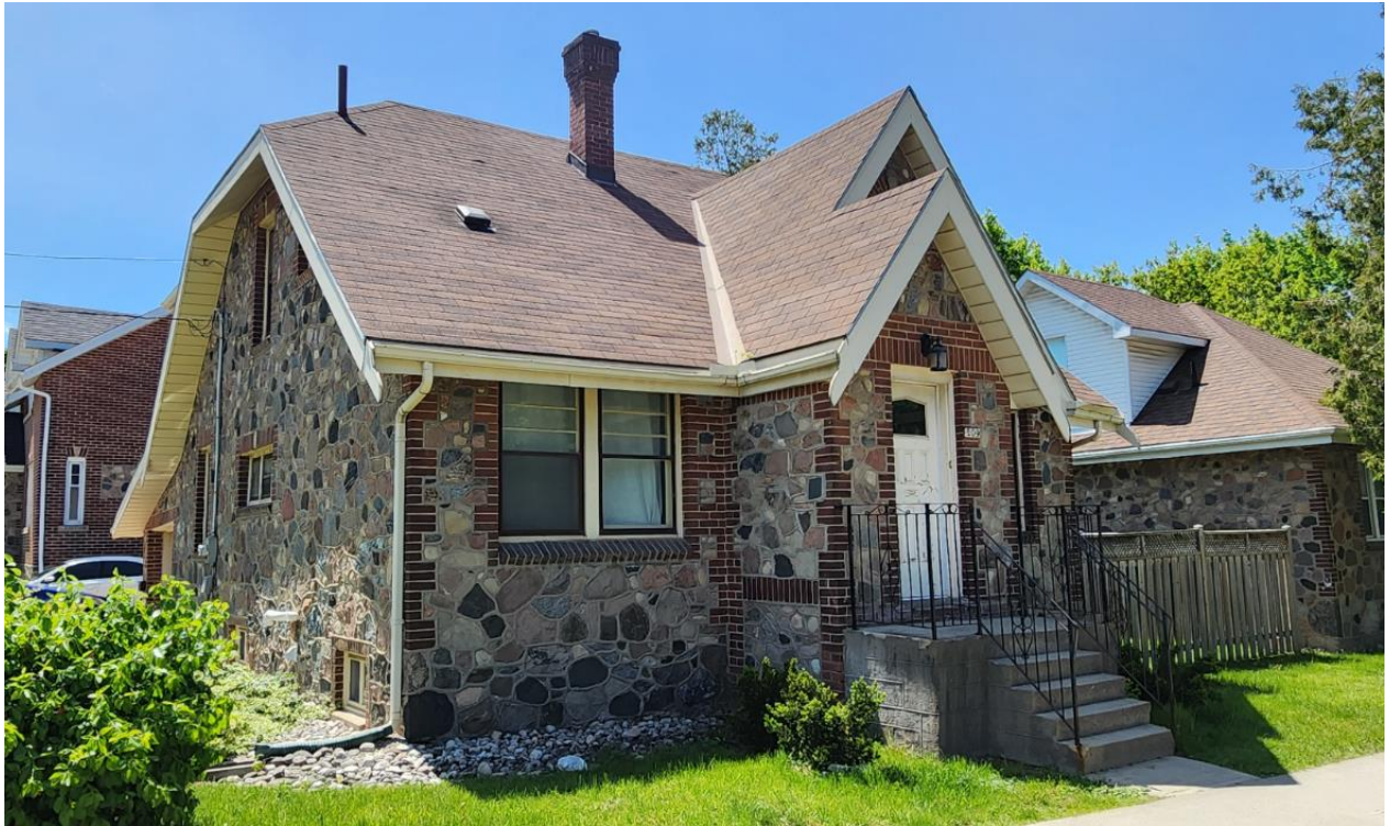
Figure 5 - 209 Gordon St, example of mixed fieldstone with brick trim construction (Photo: S. Robinson, 2023)
