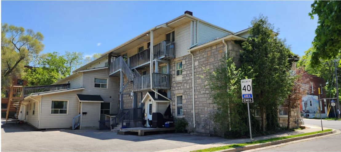
Figure 3 - 220 Gordon St, rear of the property viewed from north. (Photo: S. Robinson, 2023)
