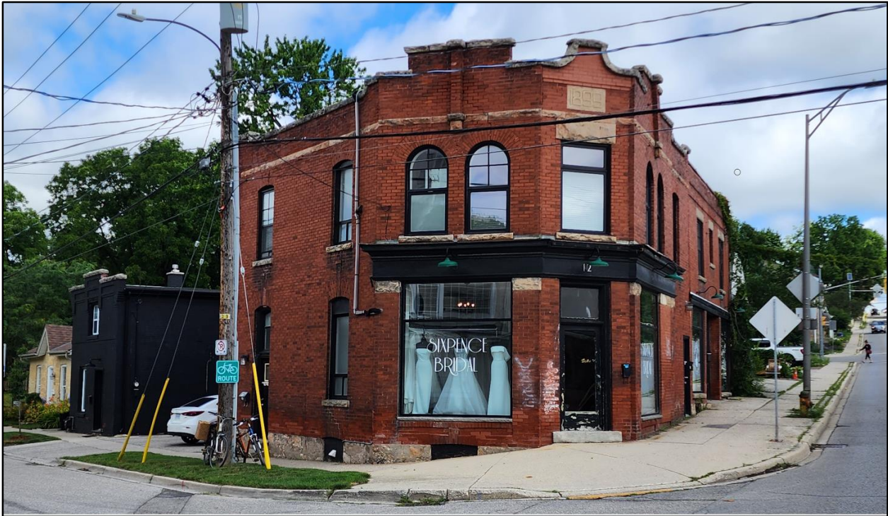
Figure 3 – 12 Eramosa Road, view from south. (Photo: S. Robinson, 2023)
