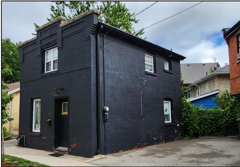
Figure 5: Stable building fronting Arthur St N. (Photo: S. Robinson, 2023)
