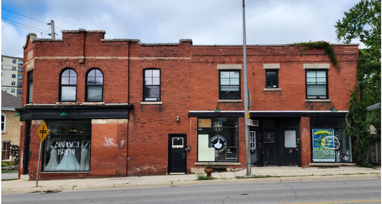
Figure 13: Eramosa Road elevation. (Photo: Sr. Robinson, 2023)
