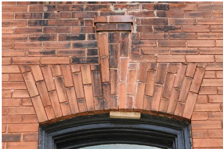
Figure 10: Brick arch over Arthur Street N door. (Photo: S. Robinson, 2023)
