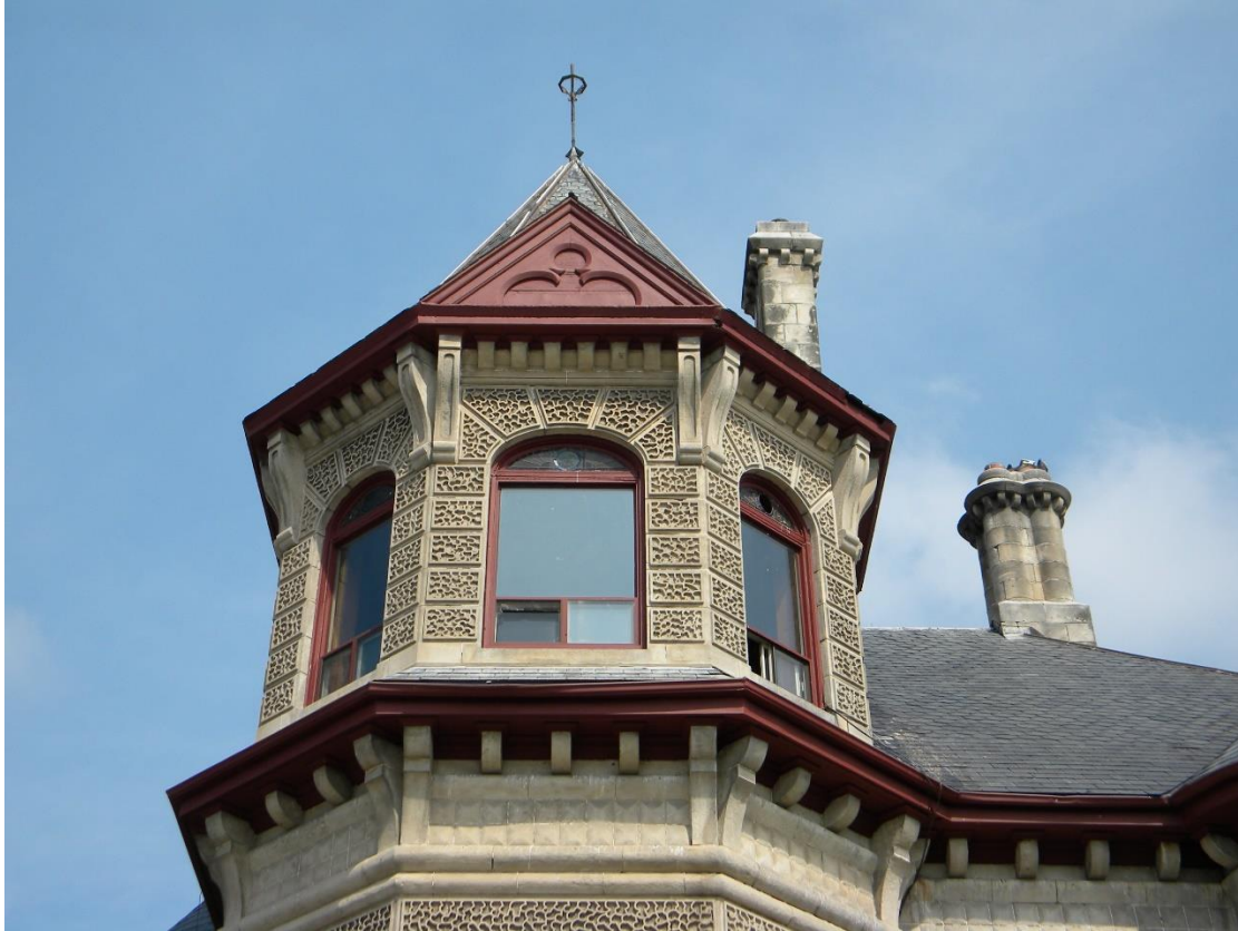
Figure 4 – 211 Silvercreek Parkway South, vermicular stone work on the tower (facing northwest) (Photo 2010 – S. Robinson)
