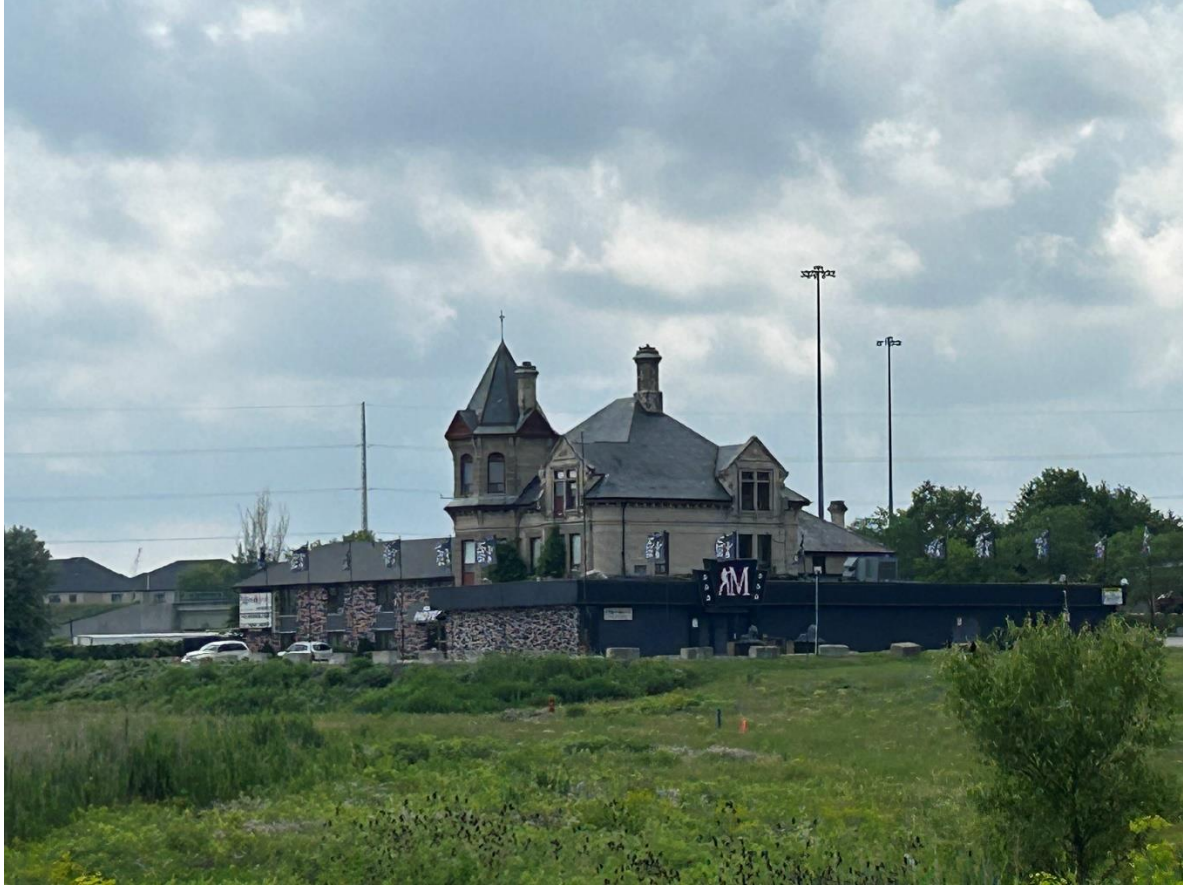
Figure 3 – 211 Silvercreek Parkway South (facing west) (Photo 2023 – V. Nagy)
