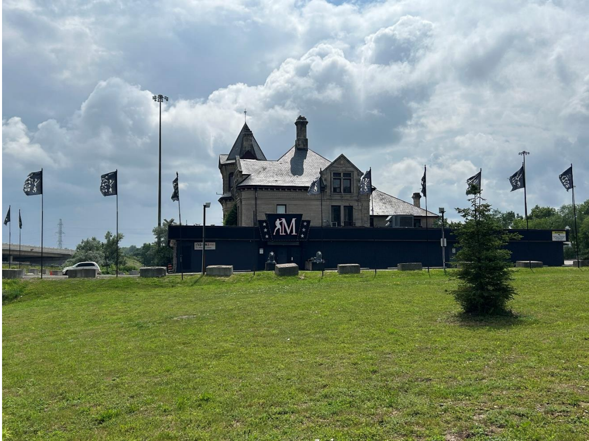
Figure 2 – 211 Silvercreek Parkway South (facing southwest) (Photo 2023 – V. Nagy)
