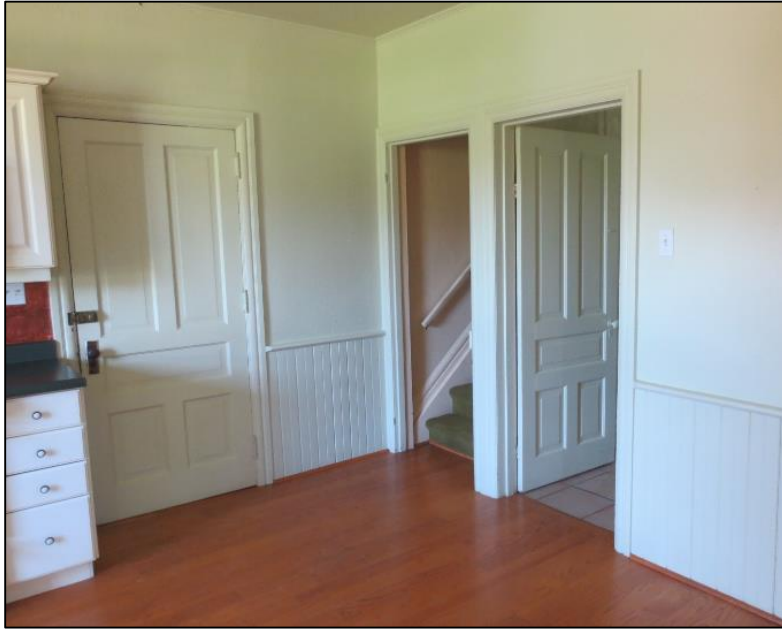
Figure 75: Photo of interior of poured-concrete farmhouse. Taken June 17, 2019, by S. Robinson.
