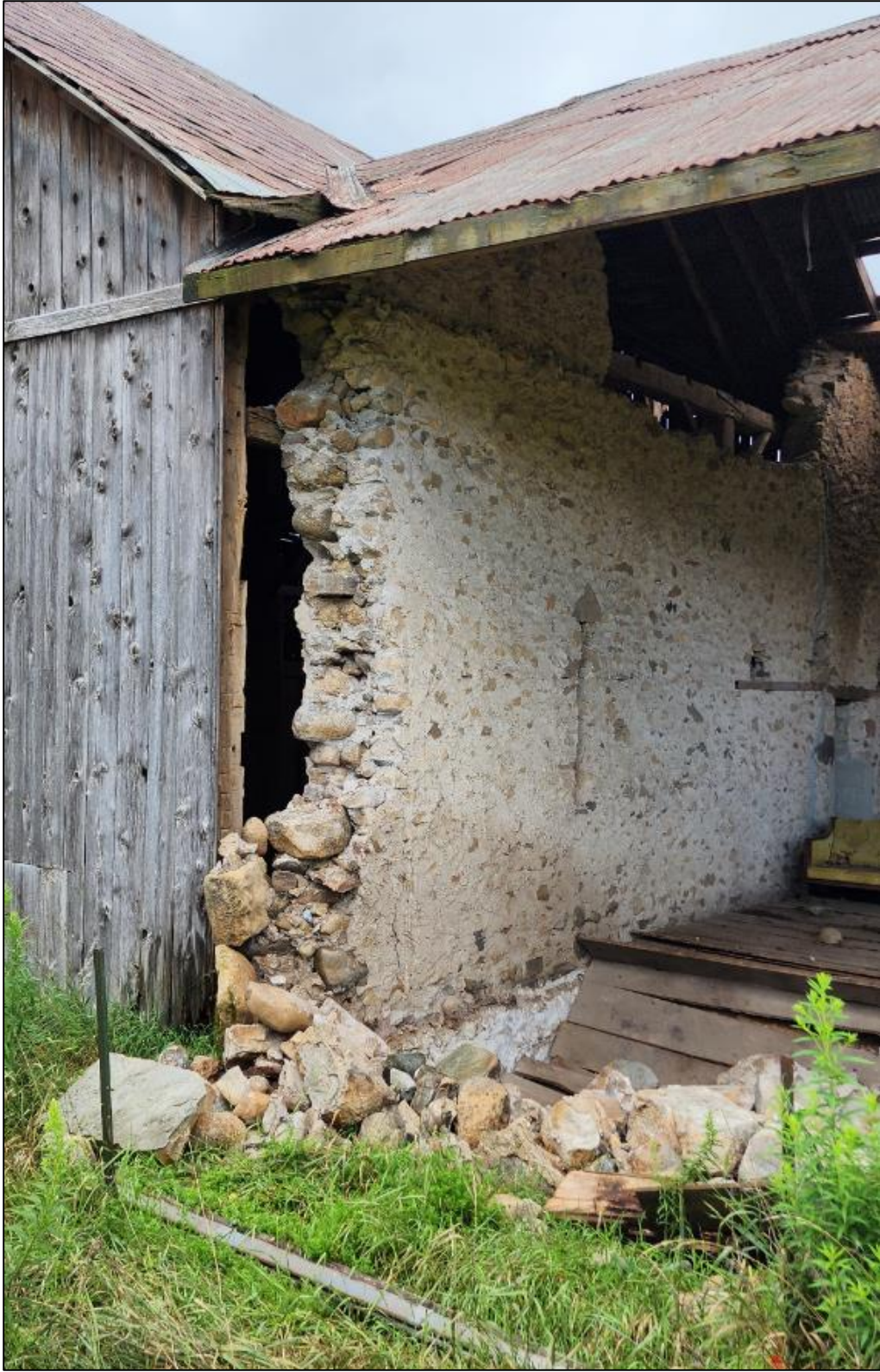
Figure 11: Photo of collapsed barn wall and compromised connecting corner. Taken July 27, 2023, by S. Robinson.
