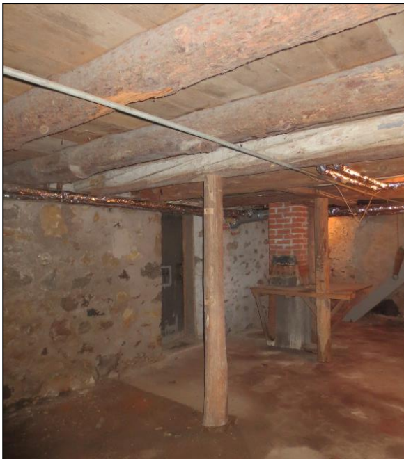
Figure 76: Photo of interior of poured-concrete farmhouse. Taken June 17, 2019, by S. Robinson.
