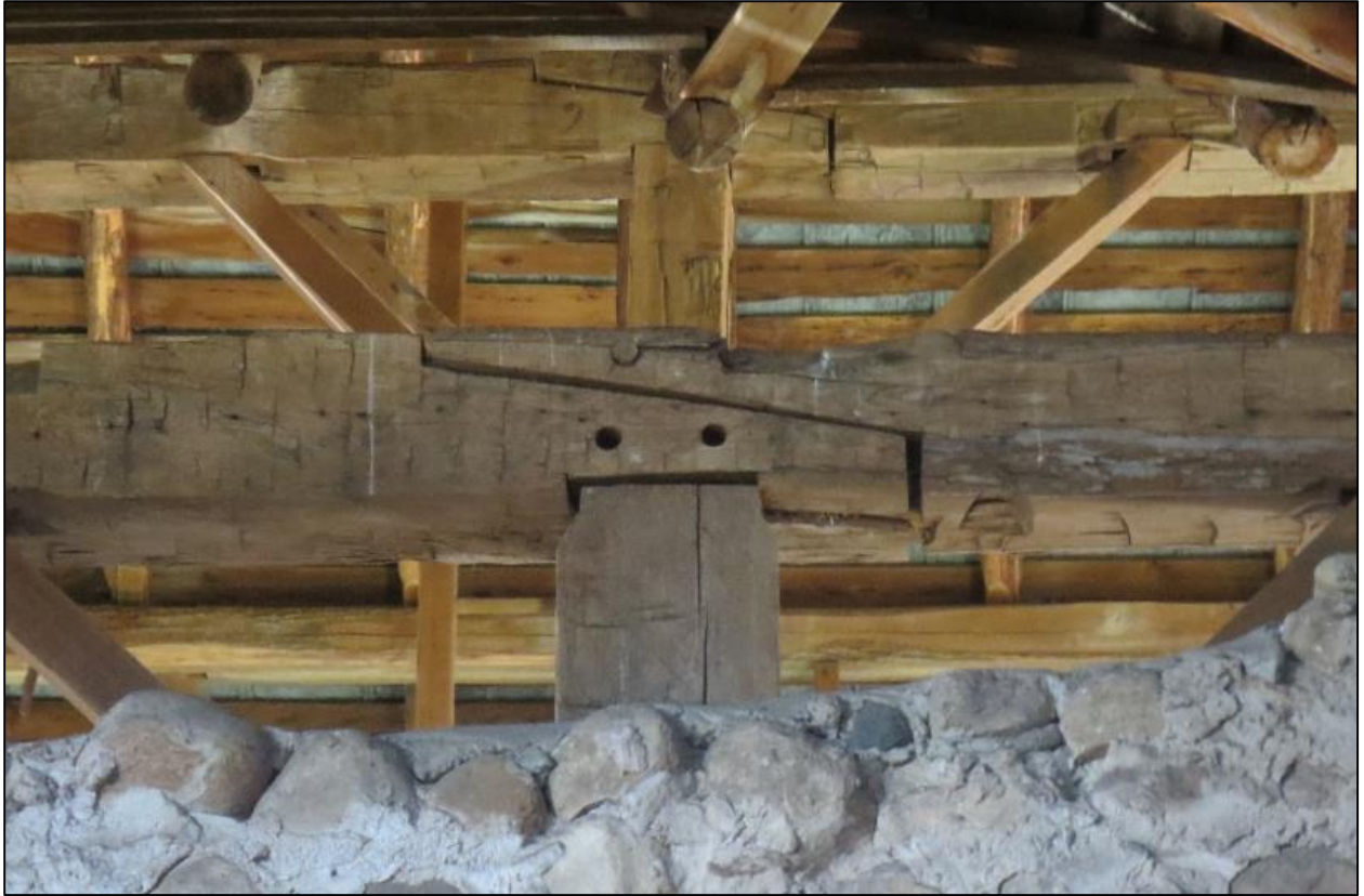
Figure 47: Photo of internal wood framing. Taken June 17, 2019, by S. Robinson.
