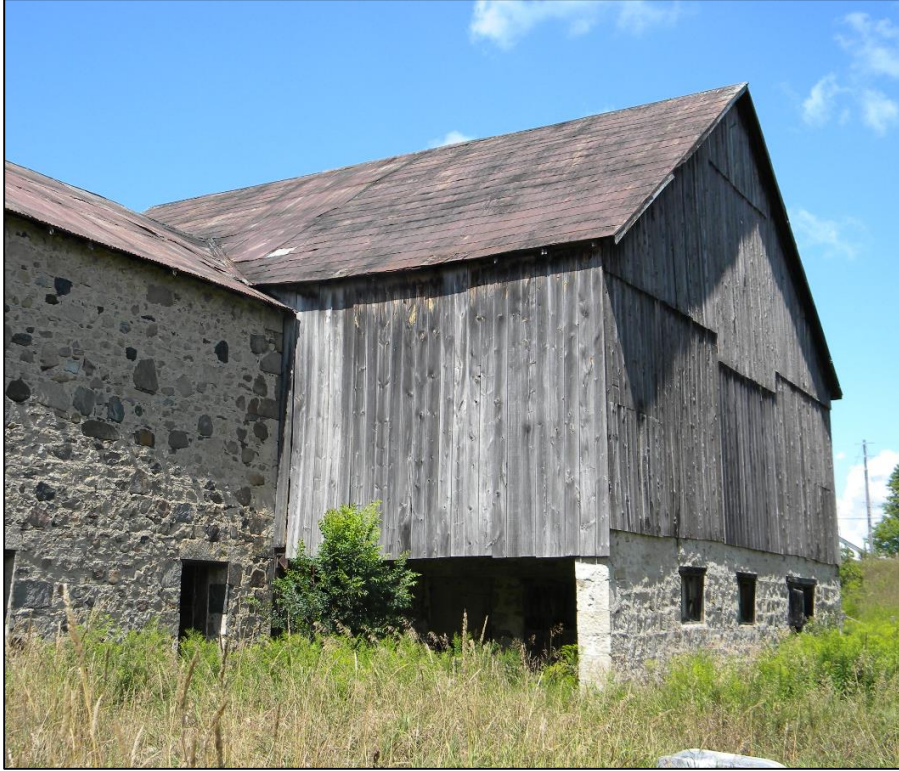
Figure 59: Photo of the stone barn and wooden addition rear exterior. Taken August 15, 2011, by S. Robinson
