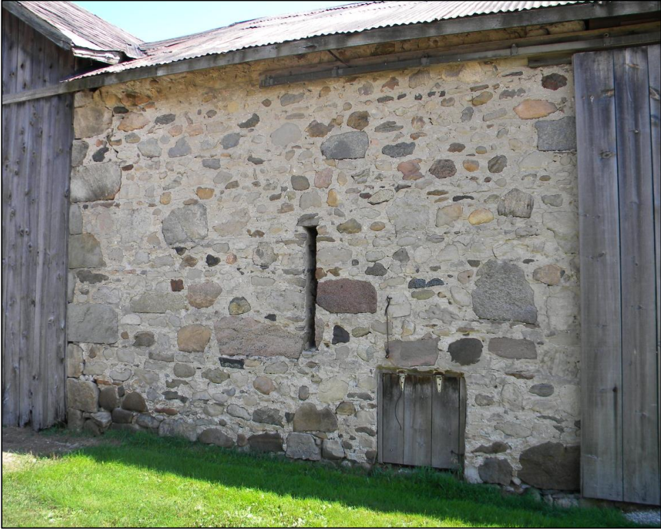
Figure 51: Photo of the stone barn exterior. Taken August 15, 2011, by S.
