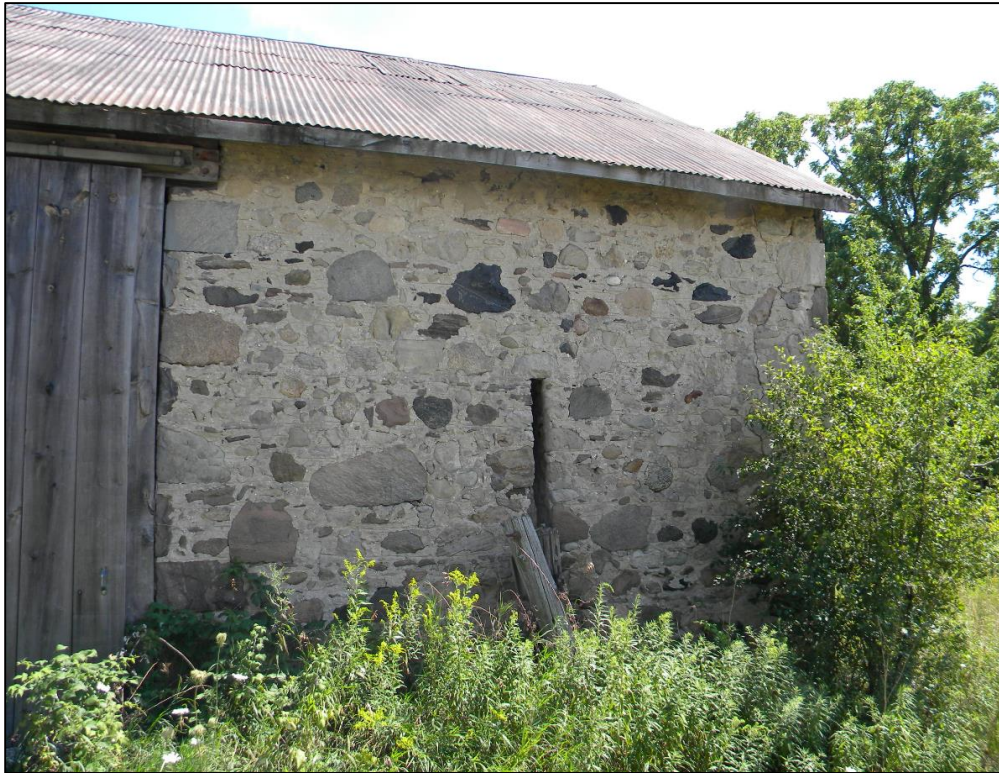
Figure 55: Photo of the stone barn exterior featuring a stone slot. Taken August 15, 2011, by S. Robinson.
