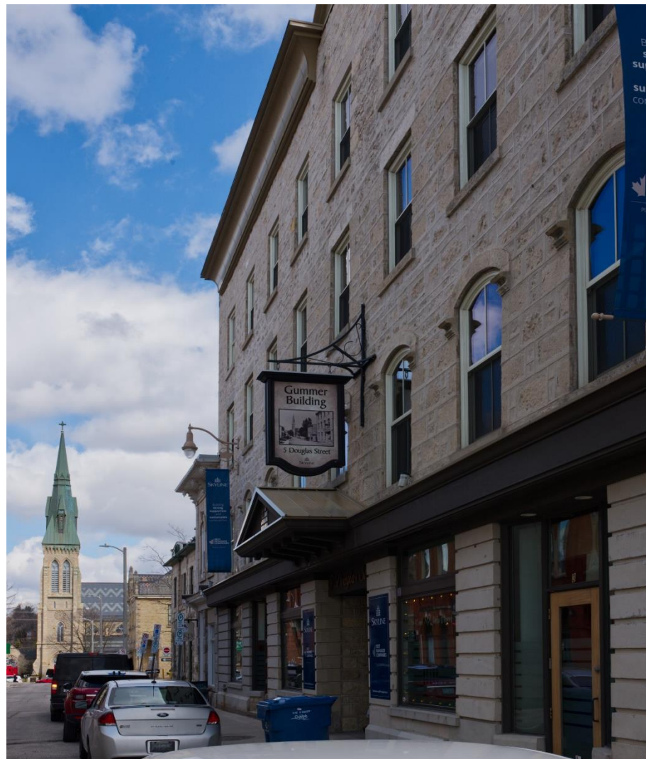
Gummer Building (Image source: Mark Steele)
