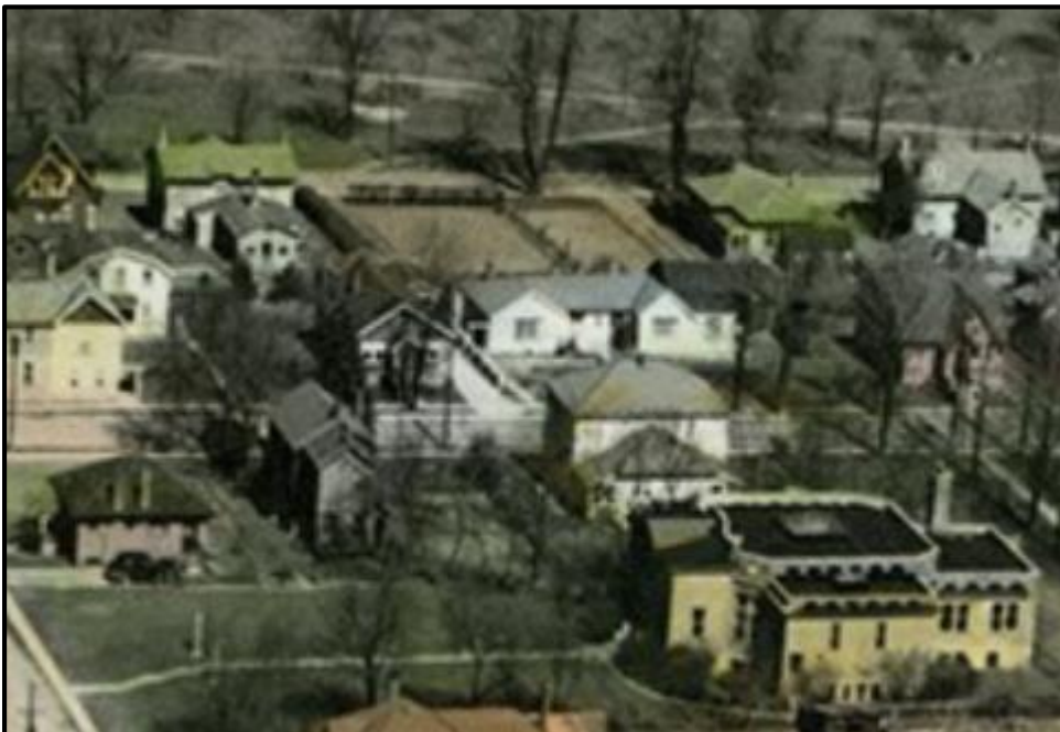
Figure 6: 1948 Aerial photograph of subject property
