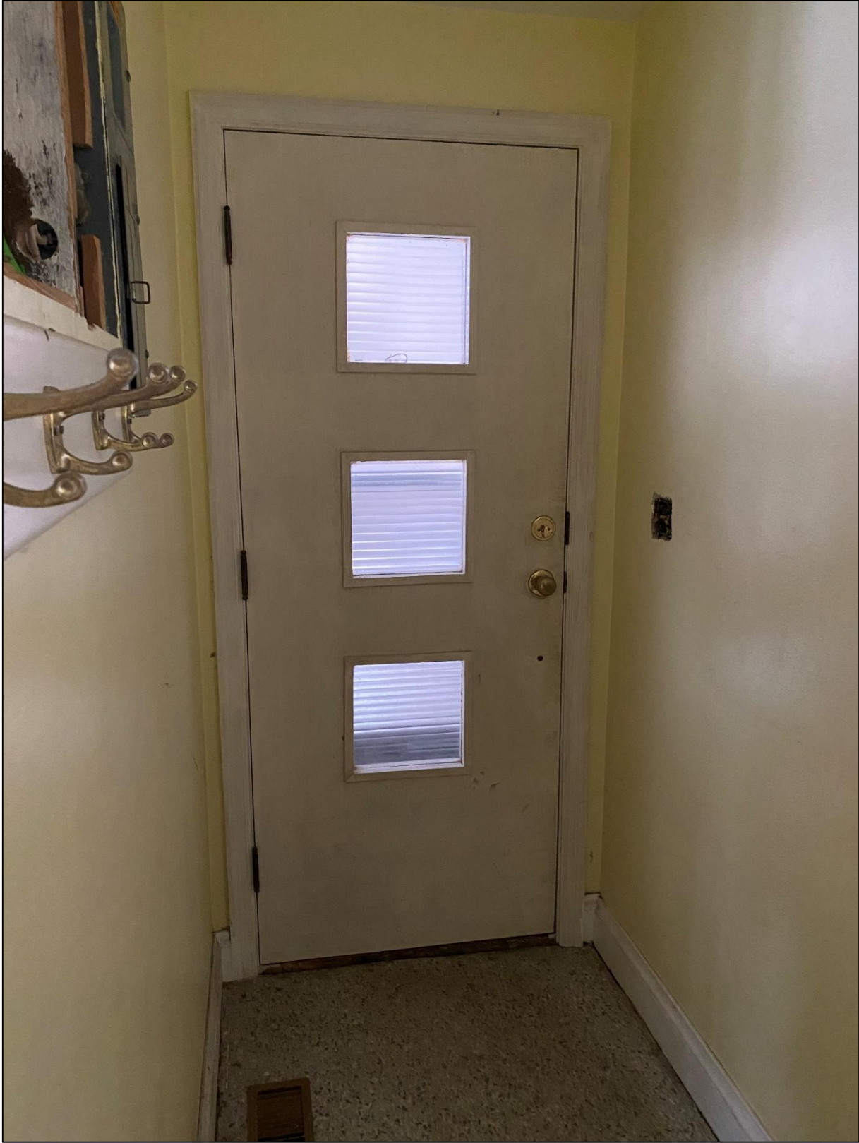
Figure 5: Interior view of the front door
