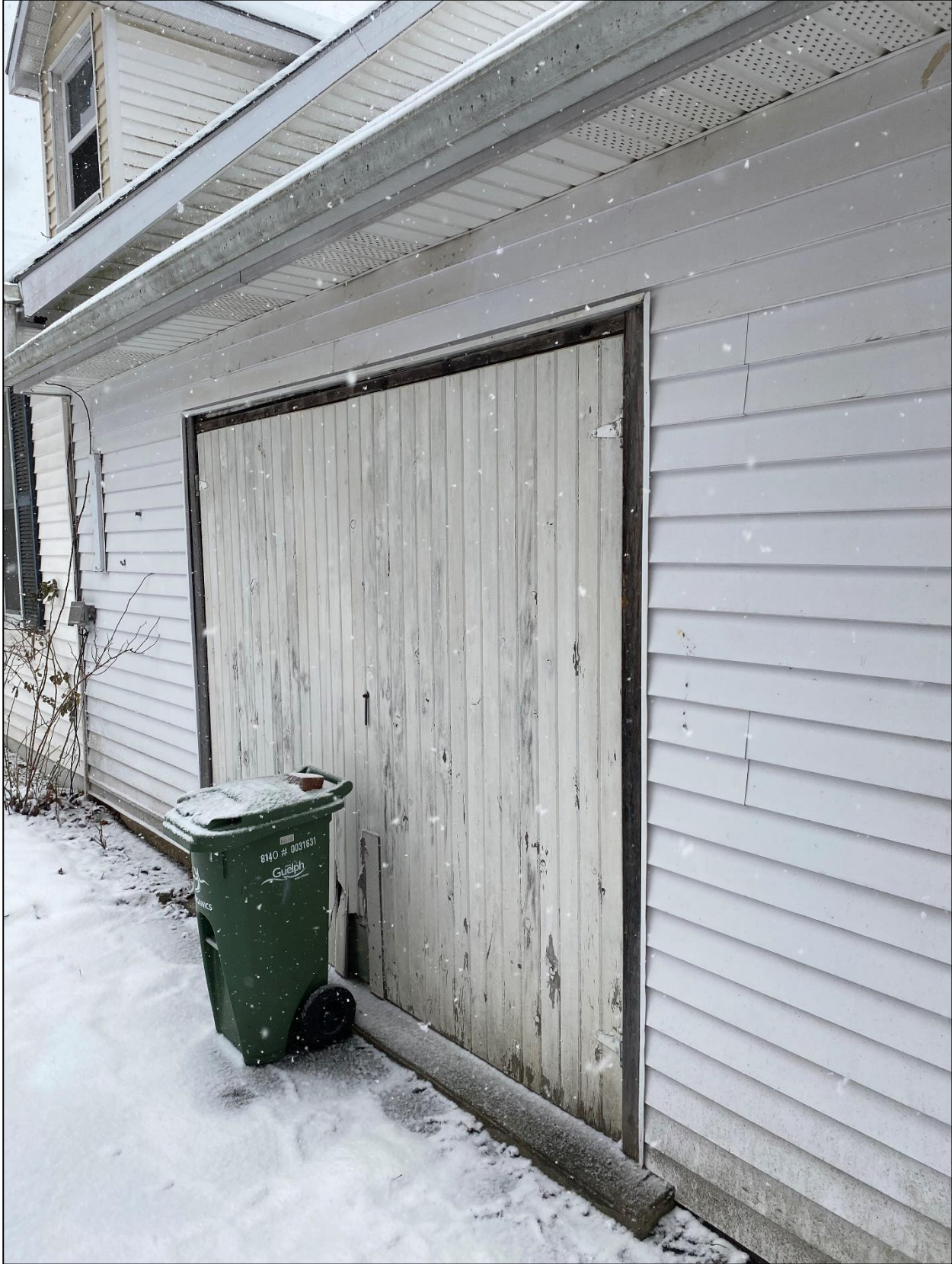
Figure 3: Close-up of the garage door
