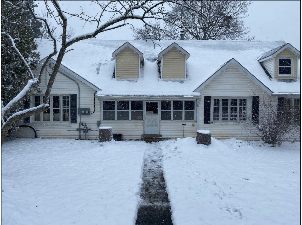
Figure 1: Front facade of the house facing Southeast
