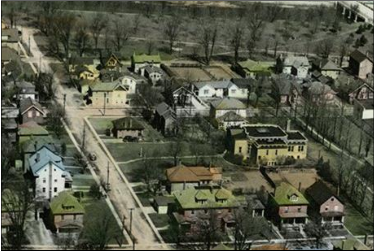
Figure 11: colour aerial photo c. 1948. GCM 160039
