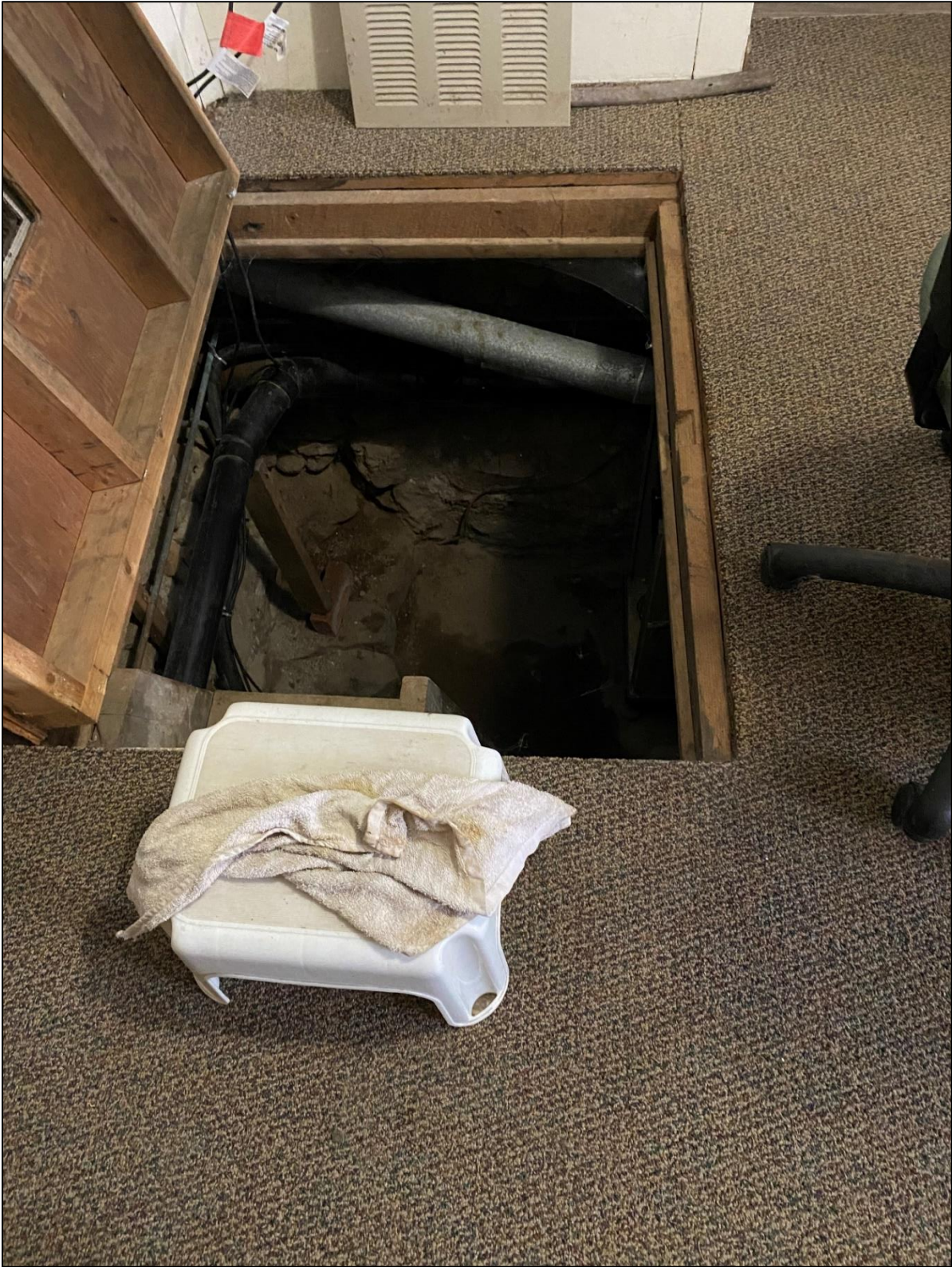
Figure 9: View into the basement from the first floor
