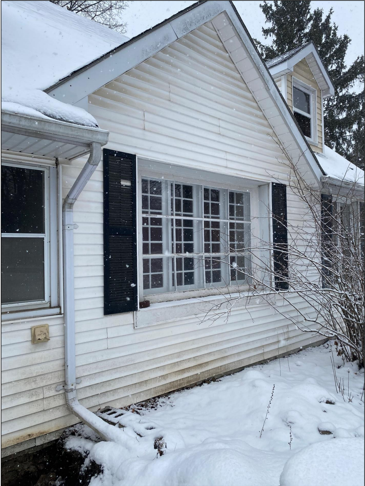
Figure 2: Close-up of the front facade
