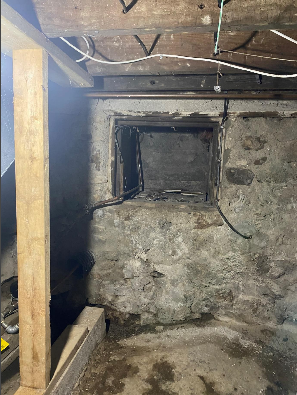
Figure 11: View of a built-in depression in the stone foundation
