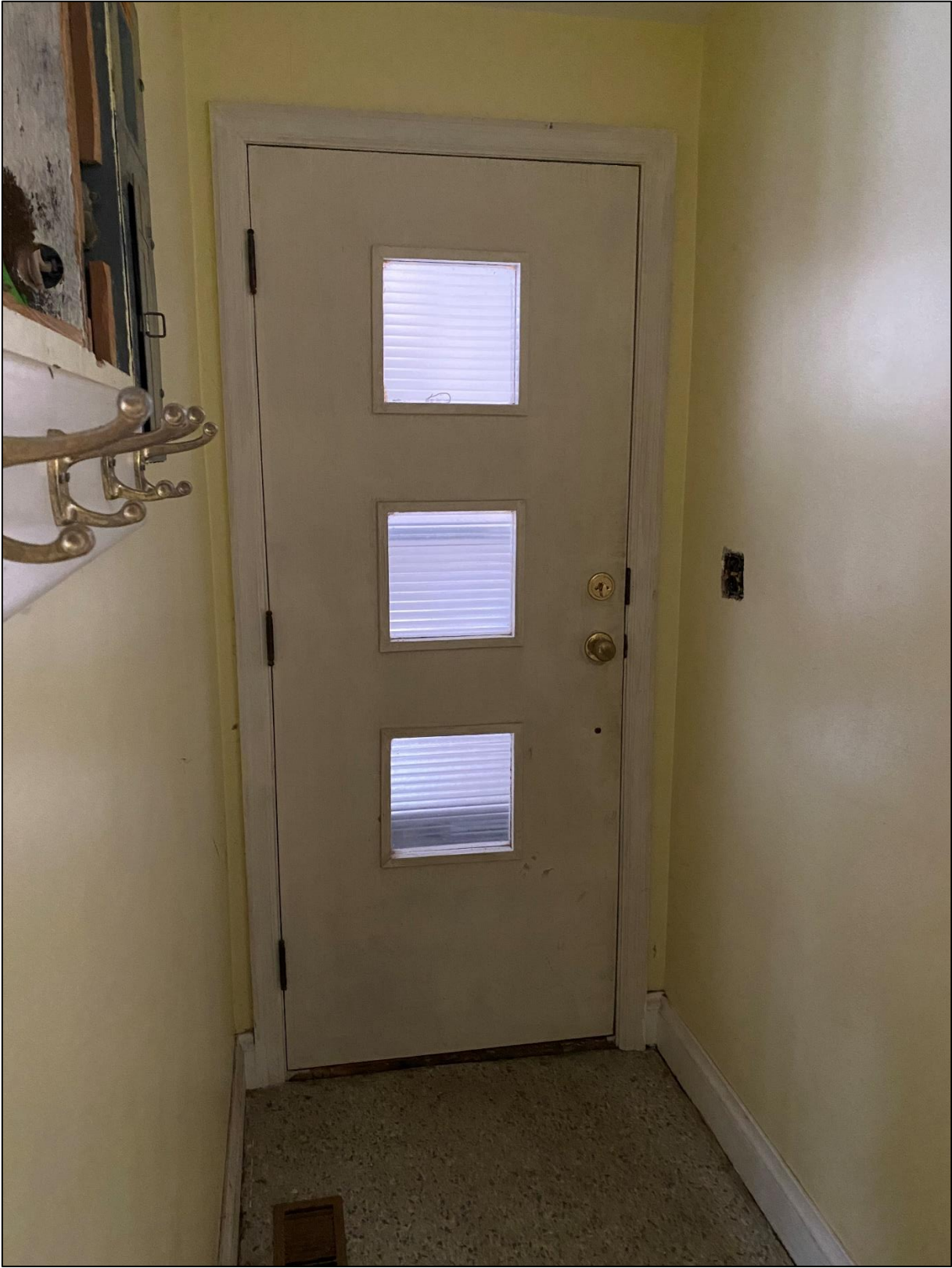
Figure 5: Interior view of the front door
