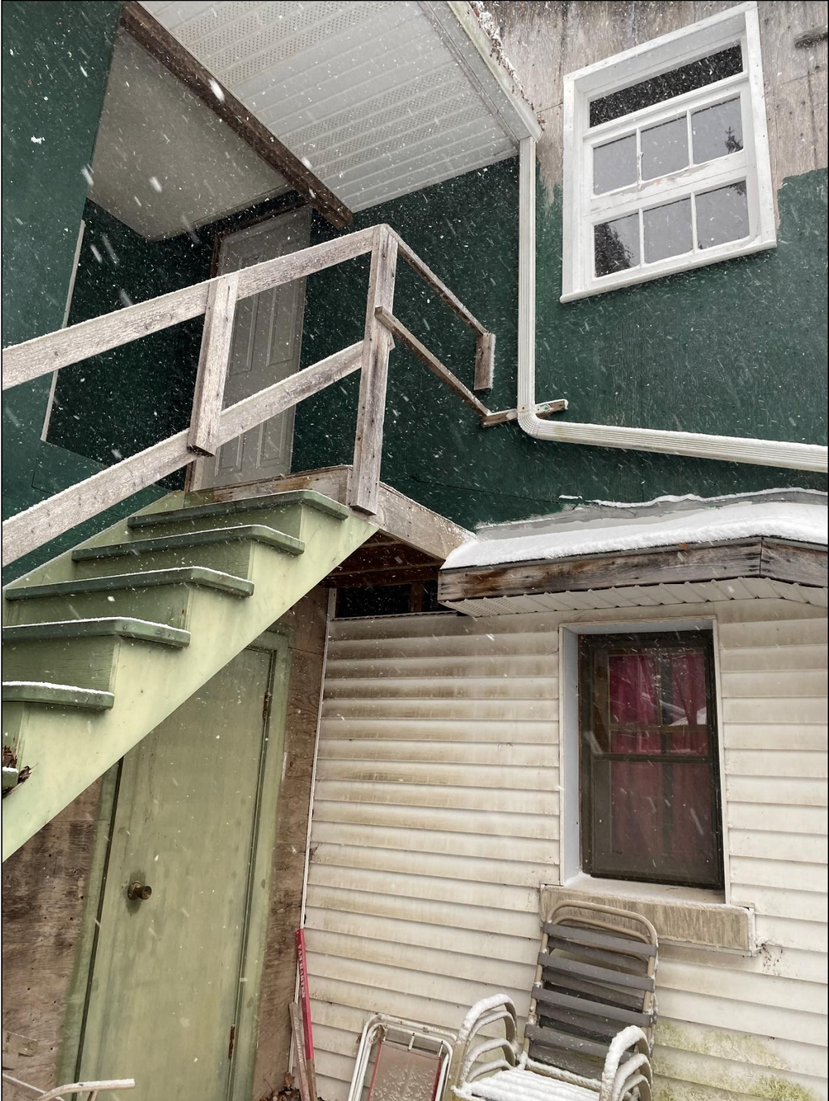
Figure 4: Rear view of the building featuring an external ground-level door, external staircase and external second floor entry.
