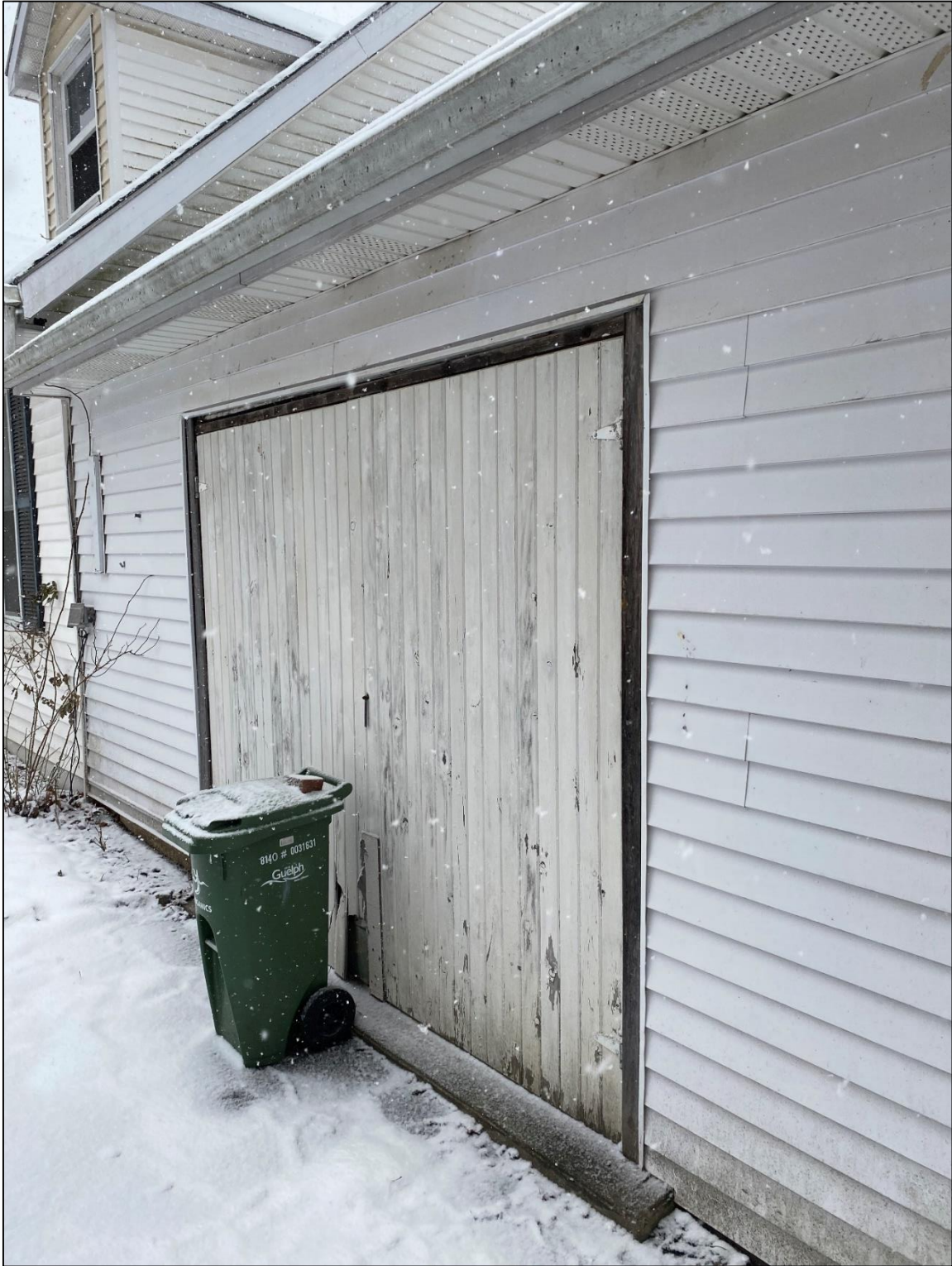
Figure 3: Close-up of the garage door
