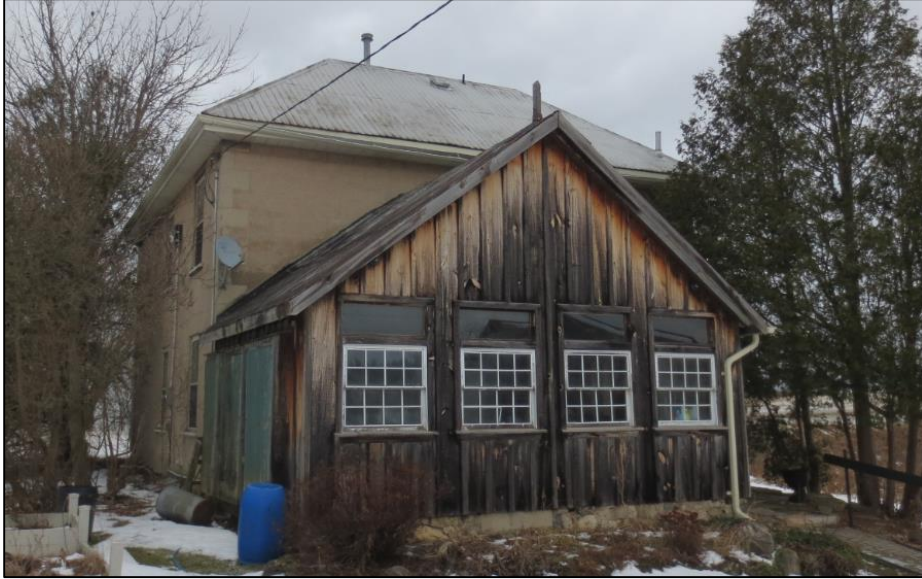
Figure 17: Image of rear exterior extension of the poured-concrete farmhouse. Taken January 24, 2019, by S. Robinson.
