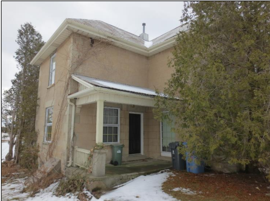
Figure 16: Image of front exterior of the poured-concrete farmhouse. Taken January 24, 2019, by S. Robinson.
