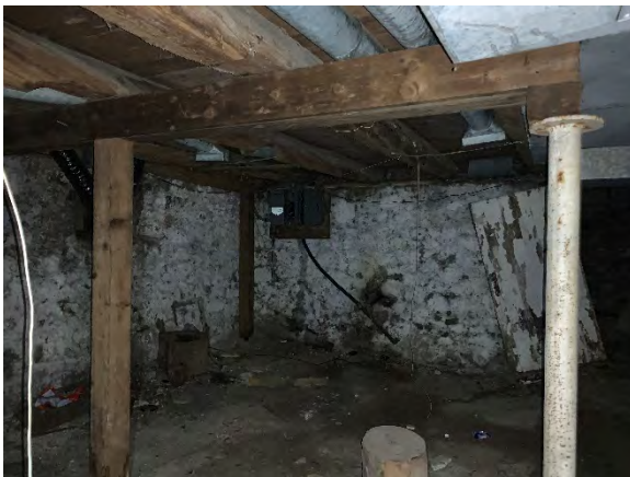
Photo 14: Typical Rubble Foundation Wall
