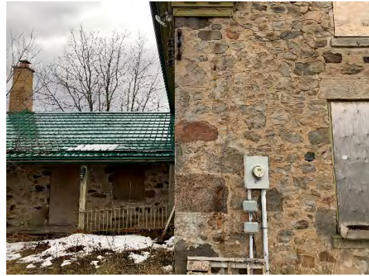
Photo 6: Typical Un-coursed Rubble Wall with Ashlar Granite Quoins
