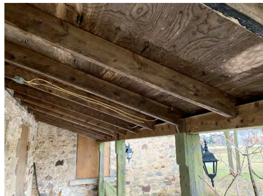
Photo 9: Underside of Covered Porch
