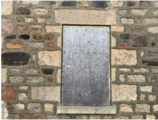
Photo 5: Typical Coursed Ashlar Wall with Dressed Jamb and Lintel
