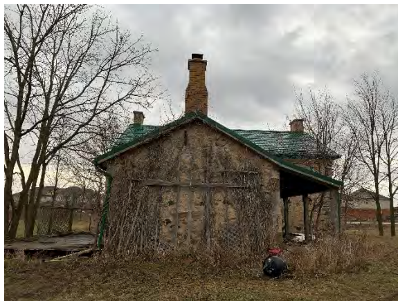
Photo 3: South Elevation (Summer Kitchen)
