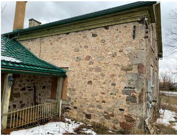
Photo 12: Typical Condition of Rubble Wall
