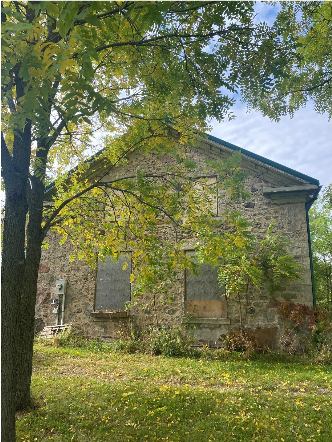
Figure 3: east facade of the James Hanlon Farmhouse
