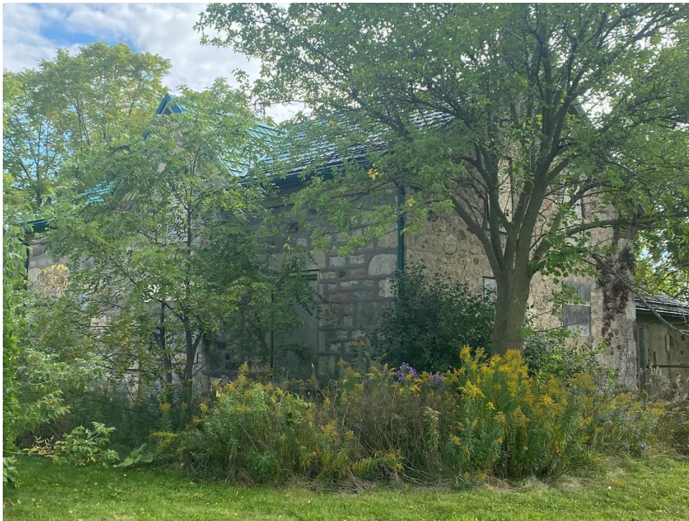
Figure 6: North and west facades of the James Hanlon farmhouse
