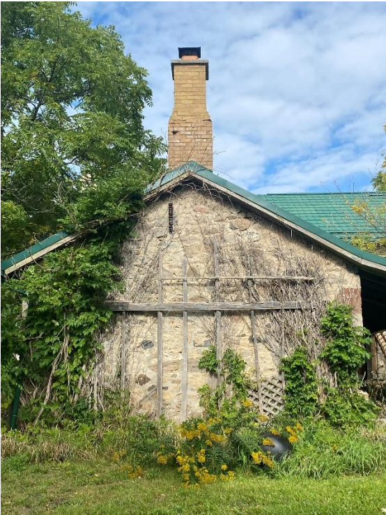
Figure 8: south facade of summer kitchen
