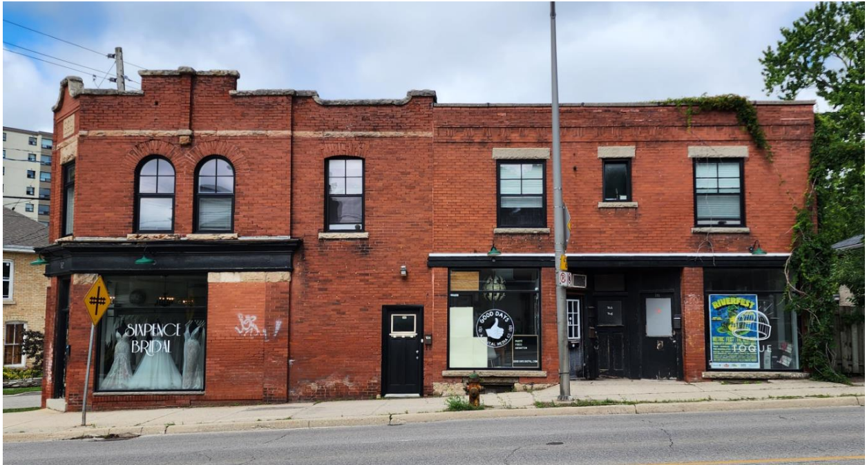
Figure 13: Eramosa Road elevation. (Photo: Sr. Robinson, 2023)
