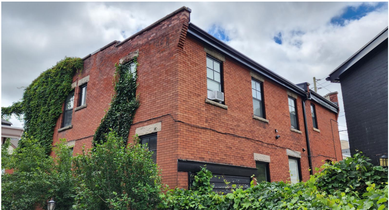
Figure 4: View of rear (north) corner. (Photo: S. Robinson, 2023)
