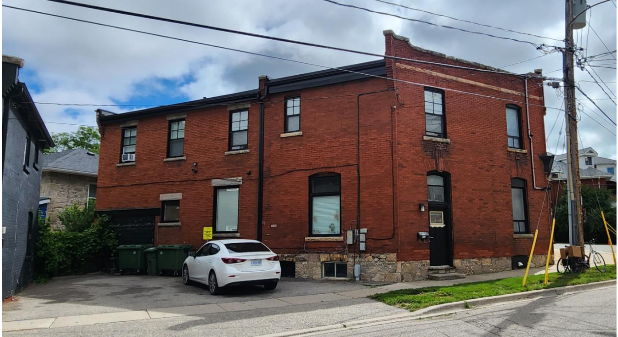
Figure 5: View of corner building from west. (Photo: S. Robinson, 2023)
