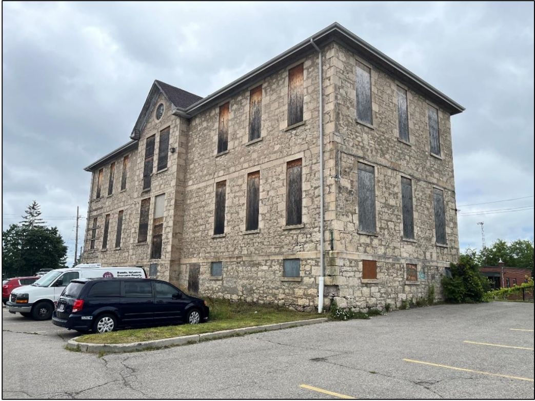
Figure 7: Southeast corner of the building
