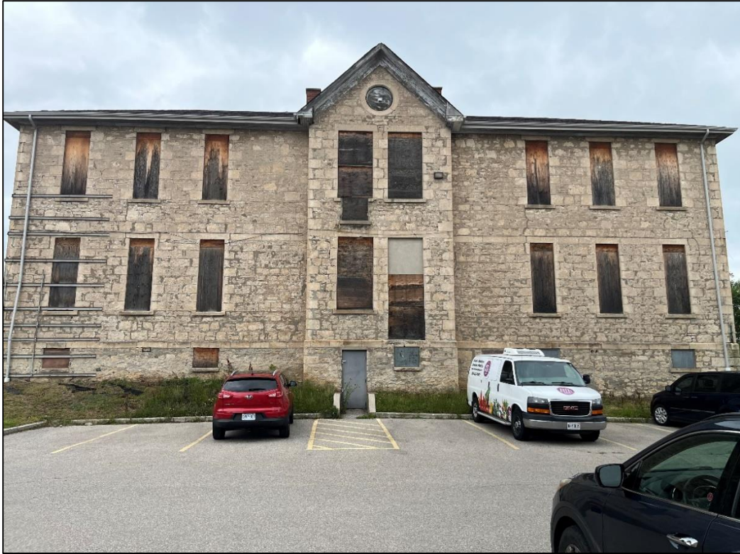
Figure 6: Southern (rear) façade of the building
