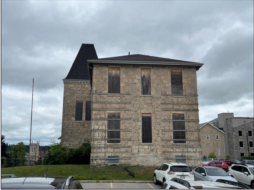
Figure 4: Western façade as viewed from Dublin Street
