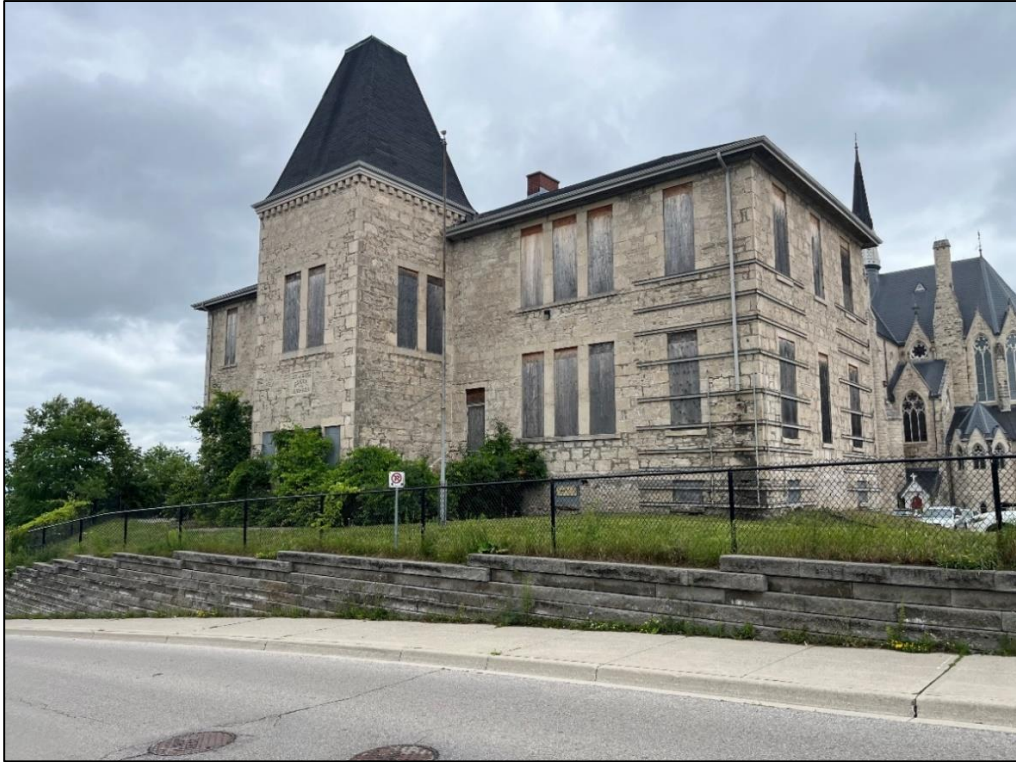
Figure 3: Northwest corner of the building viewed from Cork Street
