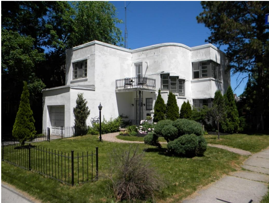
Figure 2: 49 Metcalfe viewed from the corner of Parkholm Avenue and Metcalfe Street
