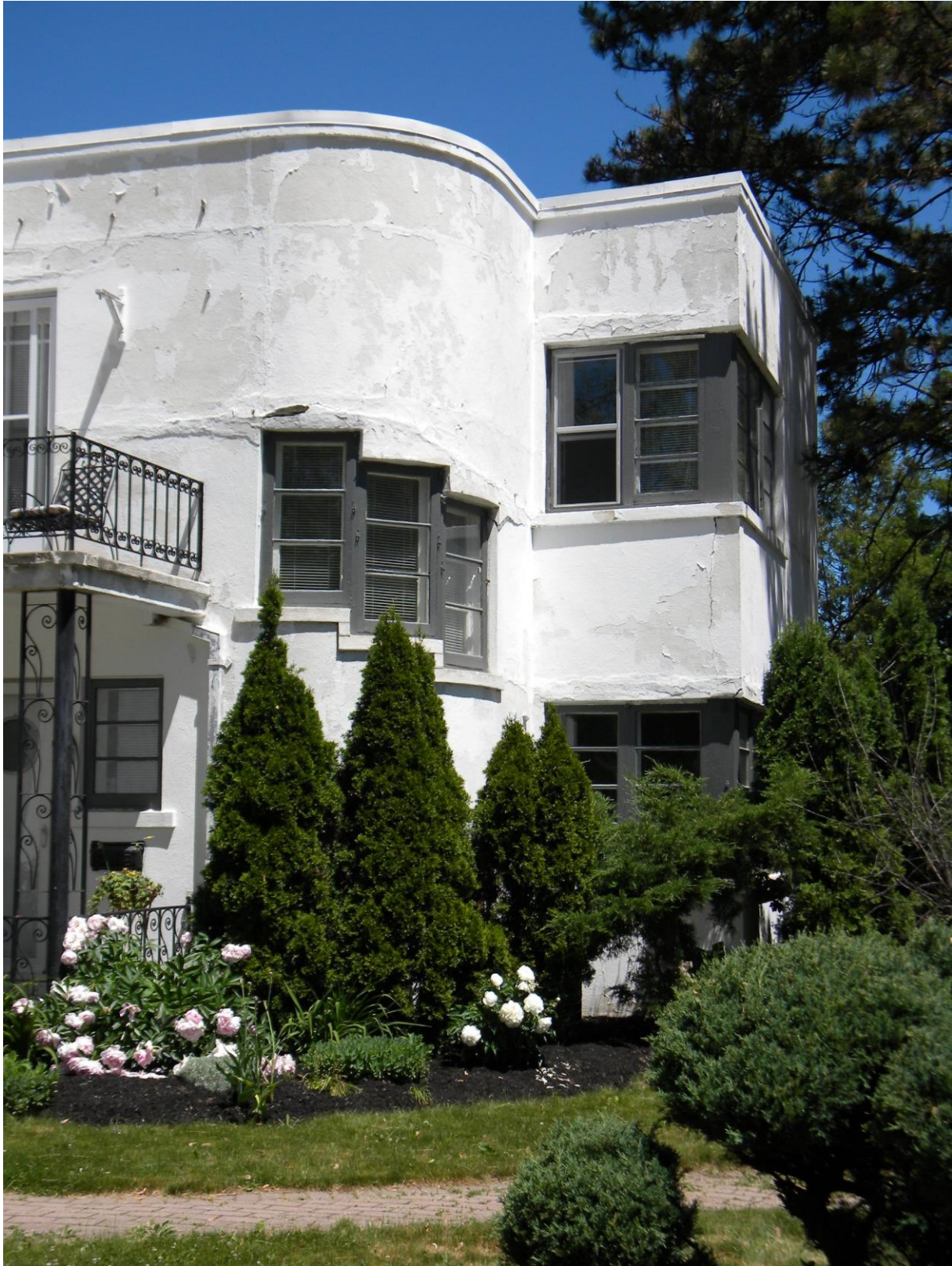
Figure 3: Curved exterior wall, stepped windows, and corner windows on the front facade of 49 Metcalfe Street
