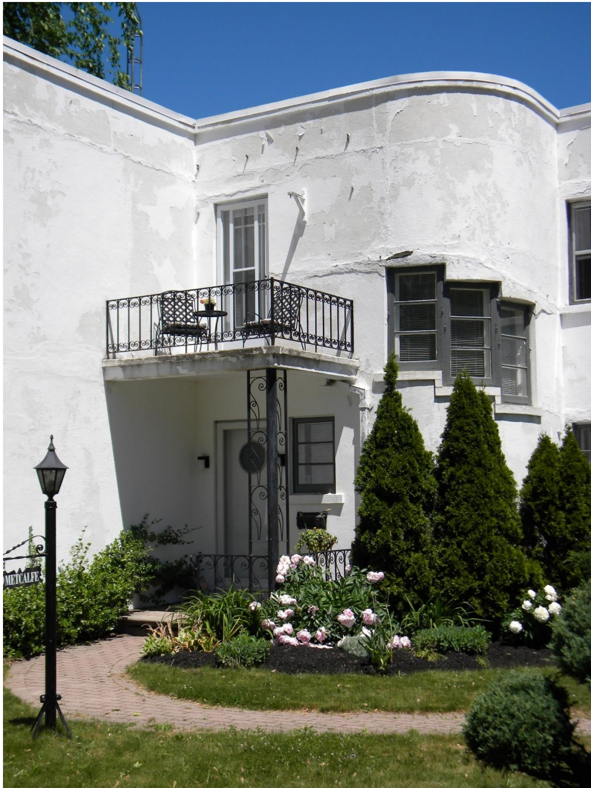
Figure 4: Front entry door with porthole window, second floor balcony with wrought iron railing, and stepped staircase window at 49 Metcalfe Street
