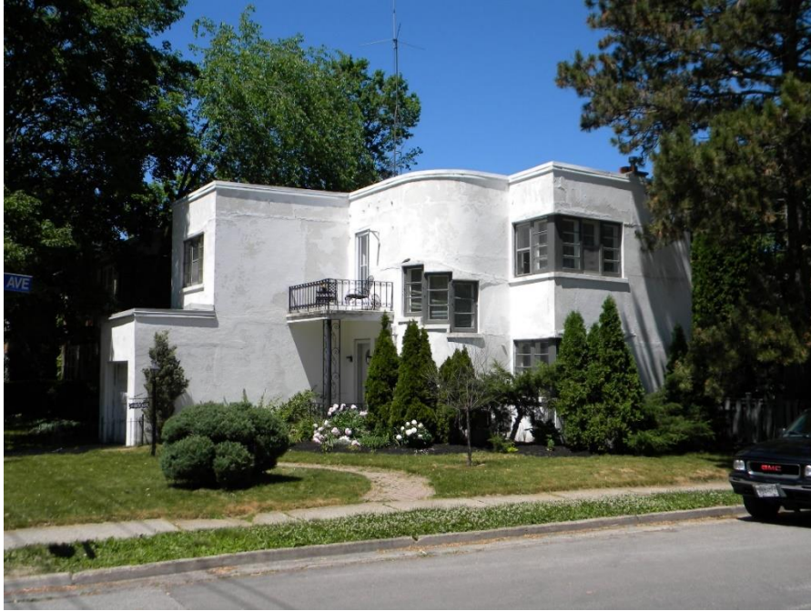
Figure 1: 49 Metcalfe viewed from across Parkholm Ave
