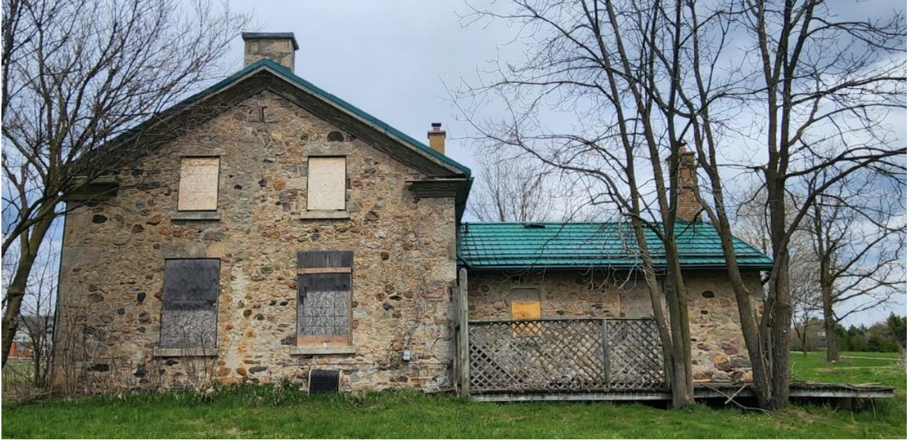
Figure 5: West facade of the Hanlon farmhouse
