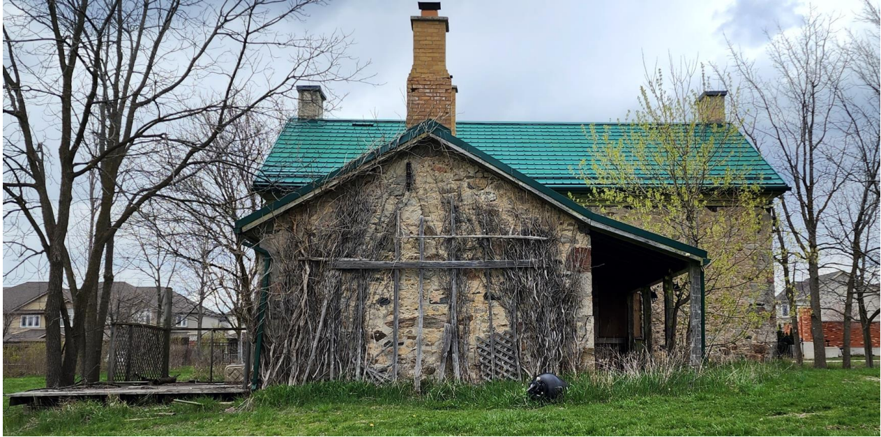
Figure 4: Rear facade of the Hanlon farmhouse
