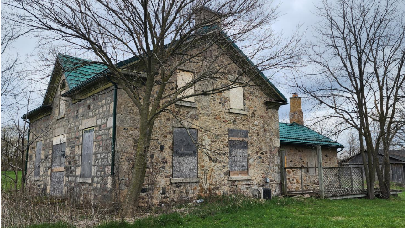
Figure 6: Northwest corner of the Hanlon farmhouse
