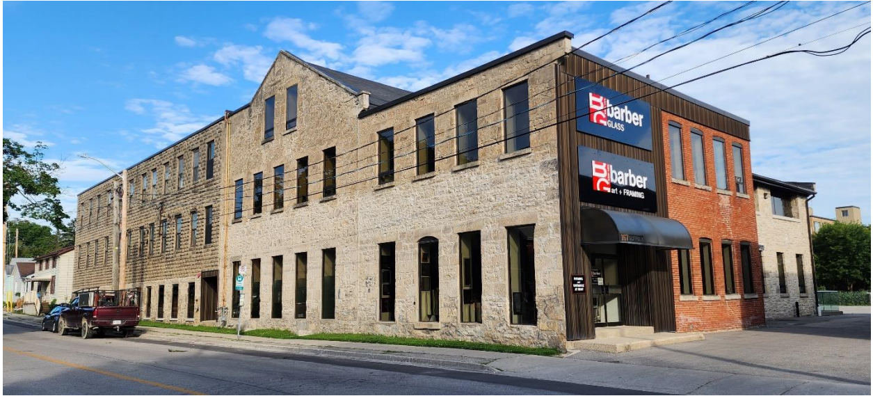
Figure 1 – Image of 167 Suffolk Street West, facing west (S. Robinson 2023).
