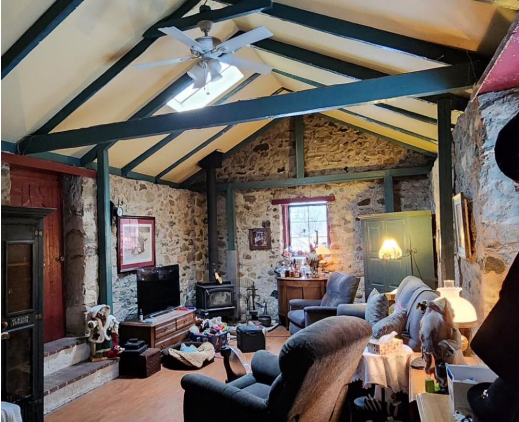
Figure 16 - Stone interior walls of east extension. (Photo S. Robinson)
