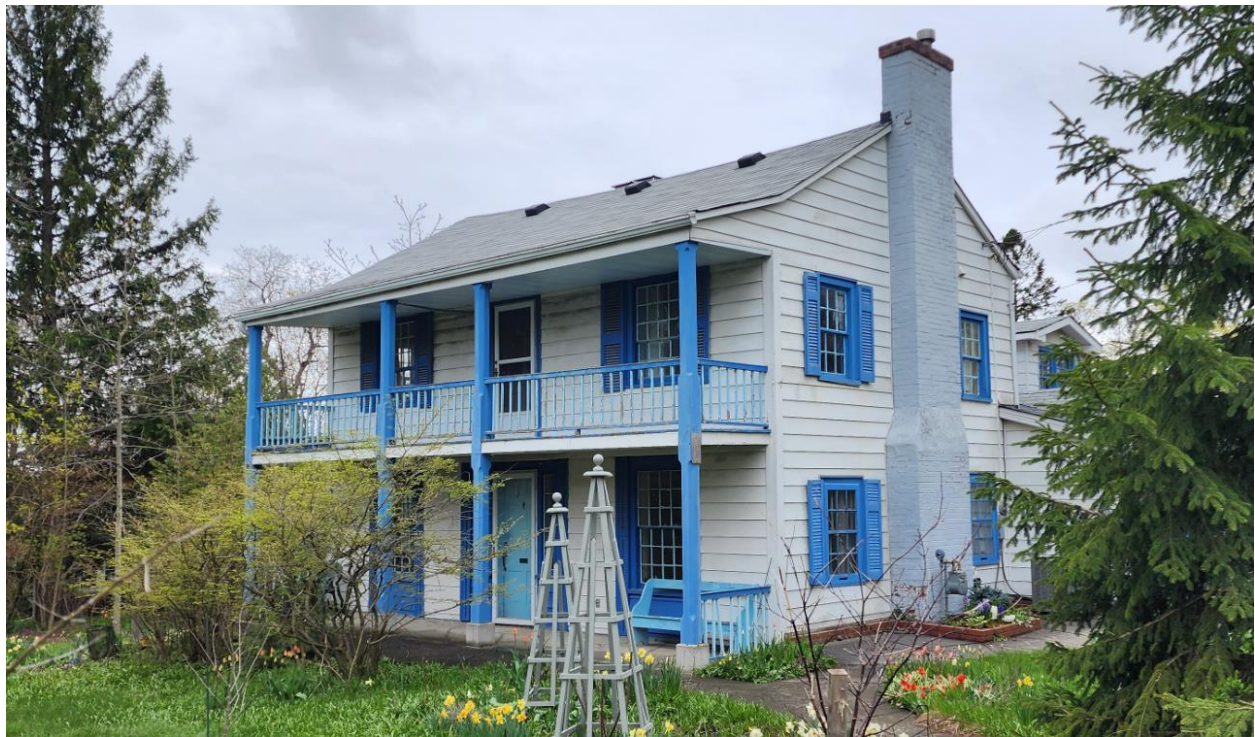
Figure 3 - View of the John Mitchell house from Queen Street. (Photo: S. Robinson, Heritage Planning, 2023)
