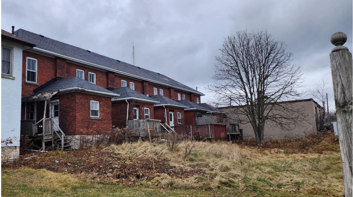
Figure 4: Rear yard of 15-23 Fountain St E (Heritage staff, 2023)
