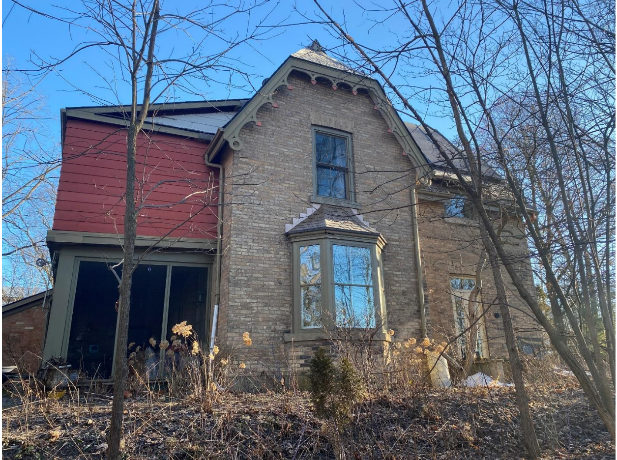
Figure 11: West elevation of 40 Spring Street (Heritage Planning Staff, 2024)
