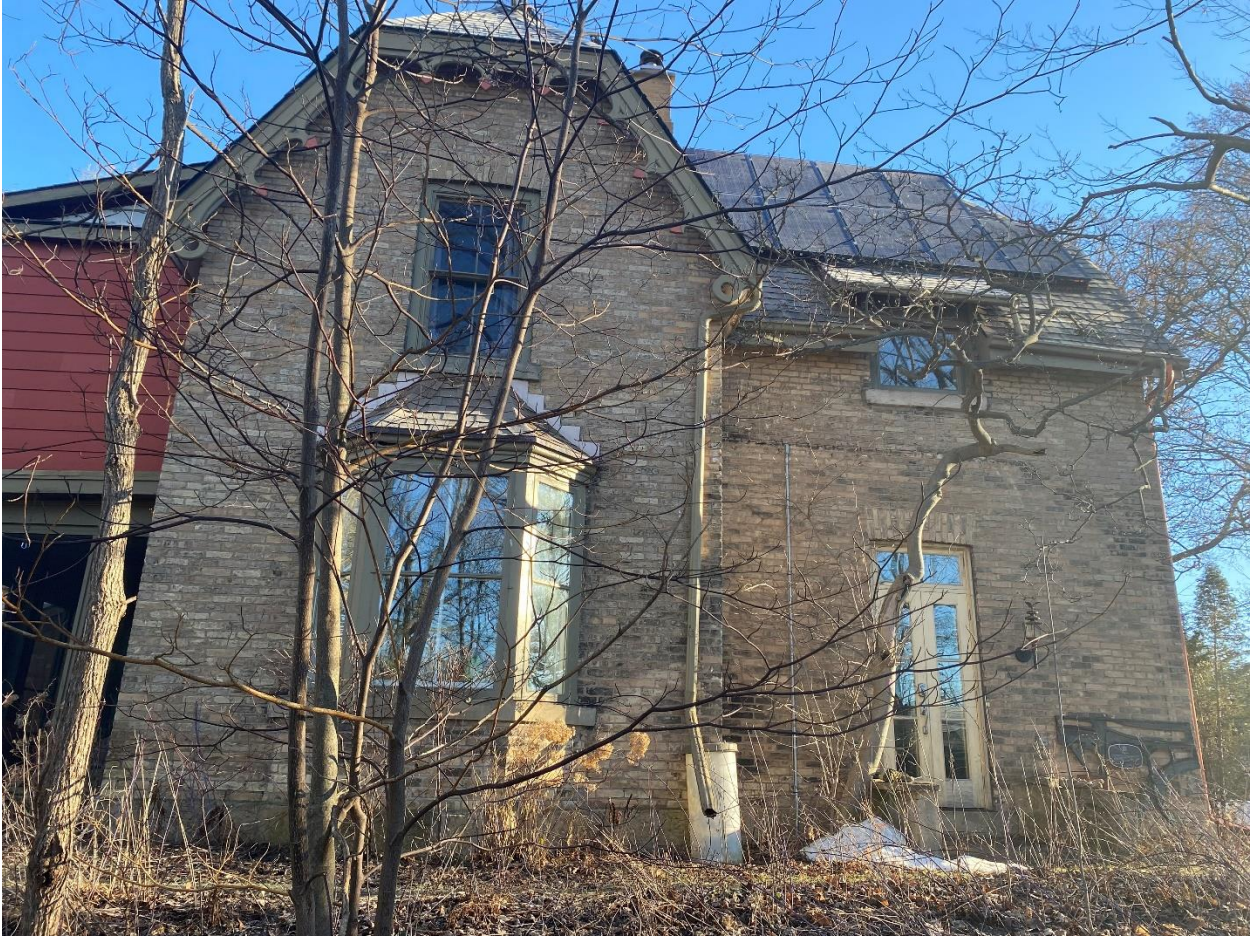
Figure 6: West elevation of 40 Spring Street (Heritage Planning Staff, 2024)
