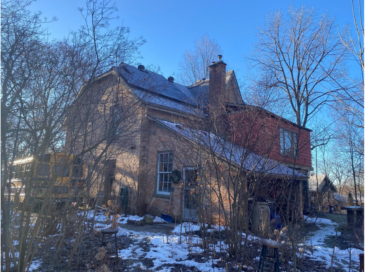
Figure 9: Northeast corner of 40 Spring Street (Heritage Planning Staff, 2024)
