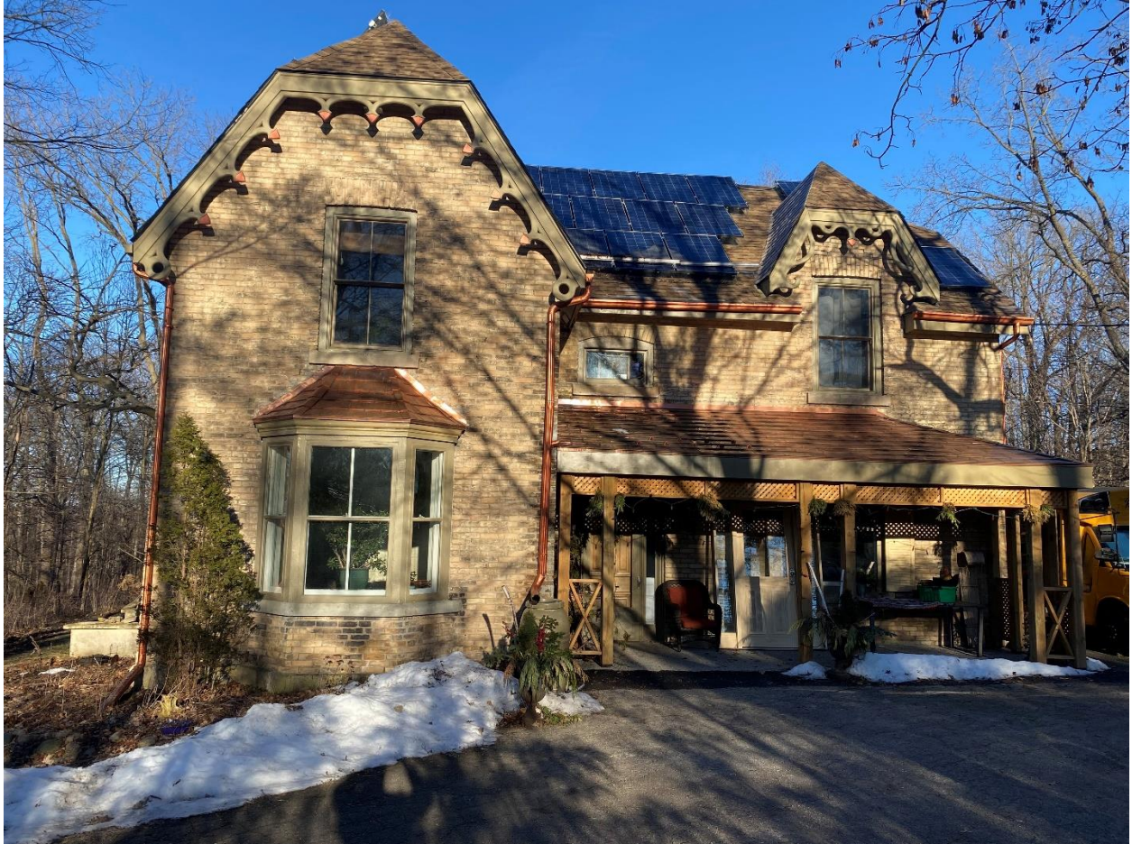
Figure 2: Facade of 40 Spring Street (Heritage Planning Staff, 2024)
