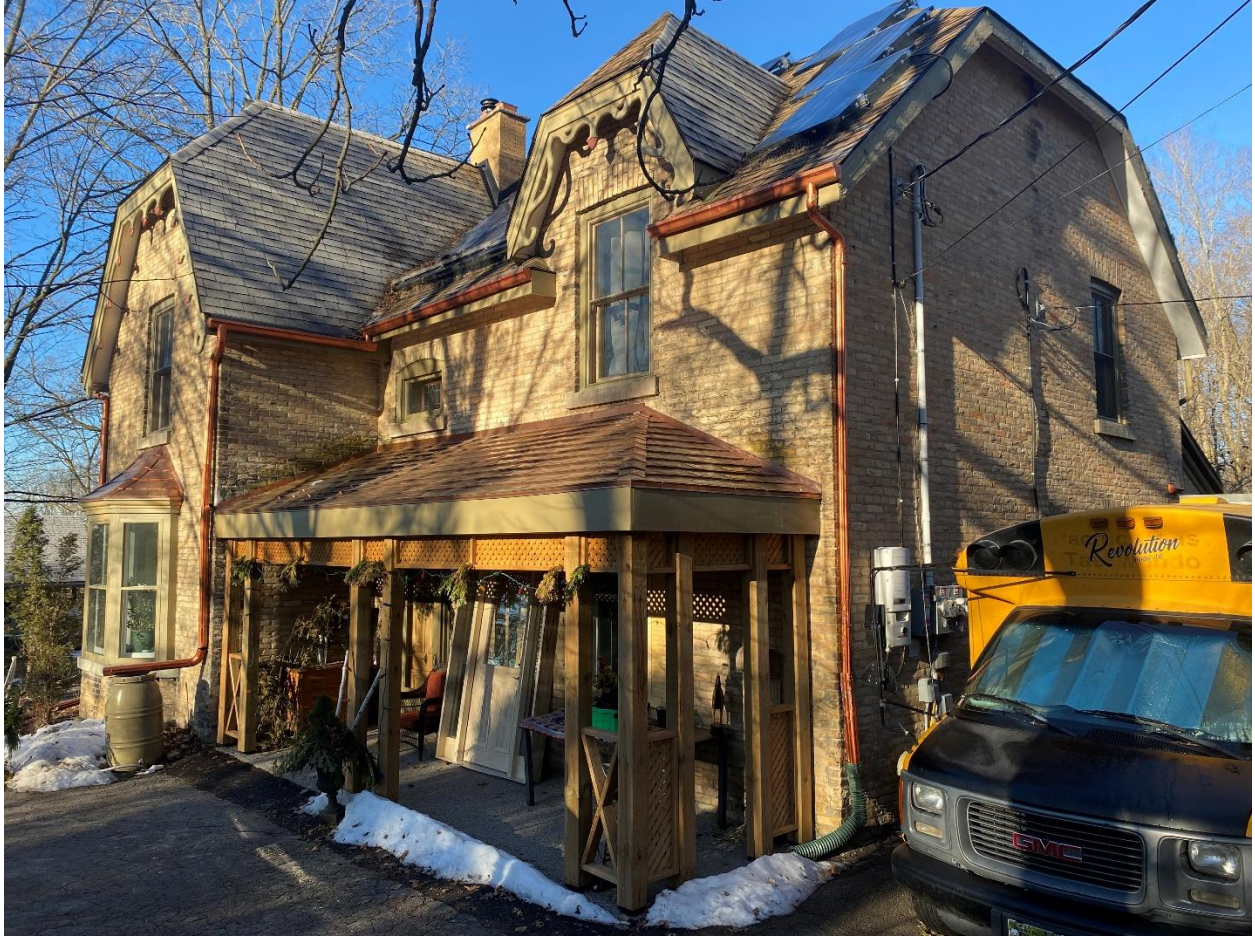
Figure 4: Southeast corner of 40 Spring Street (Heritage Planning Staff, 2024)
