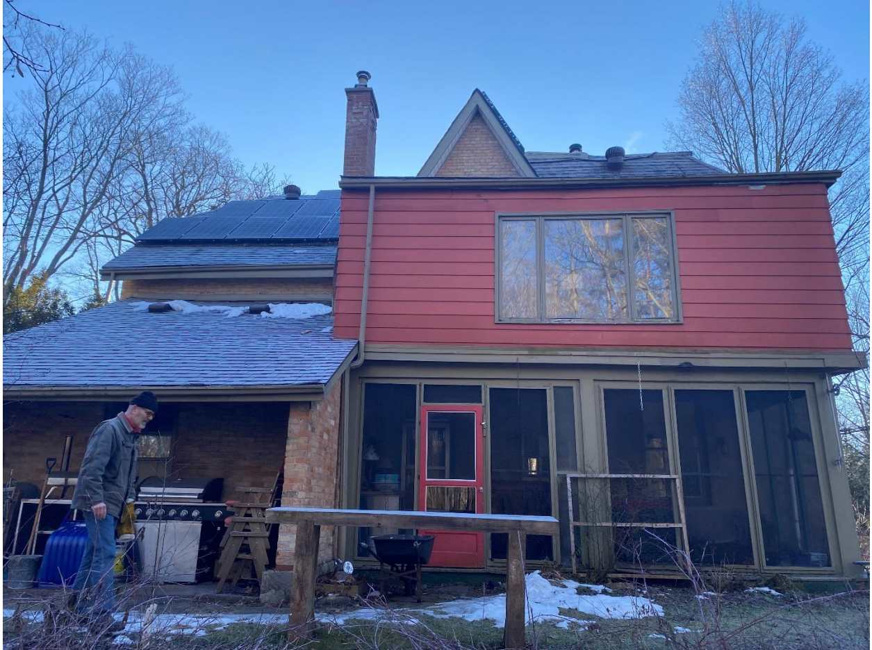
Figure 8: Rear elevation of 40 Spring Street showing the two rear additions proposed for removal (Heritage Planning Staff, 2024)
