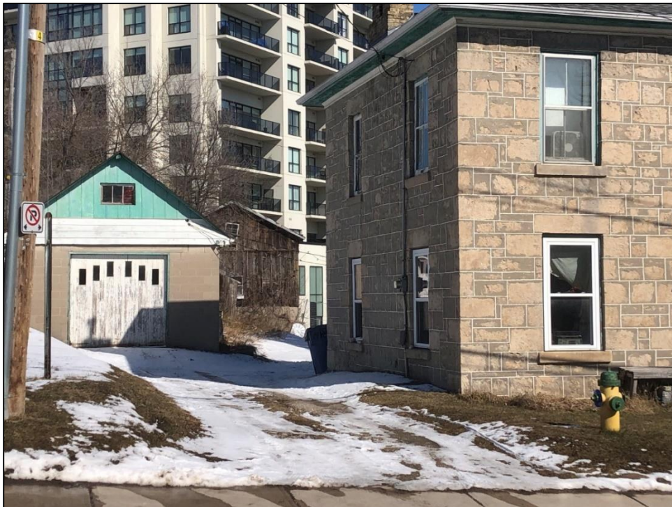
Figure 4 Photo 14 Neeve Street driveway, garage, barn, and stone house.
