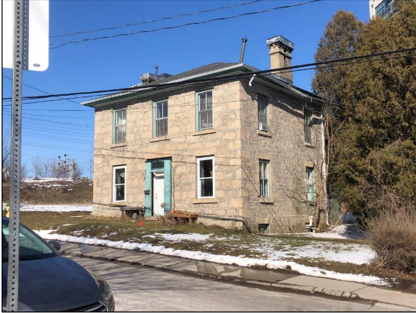
Figure 7: Photo of 14 Neeve Street Neeve Street.
