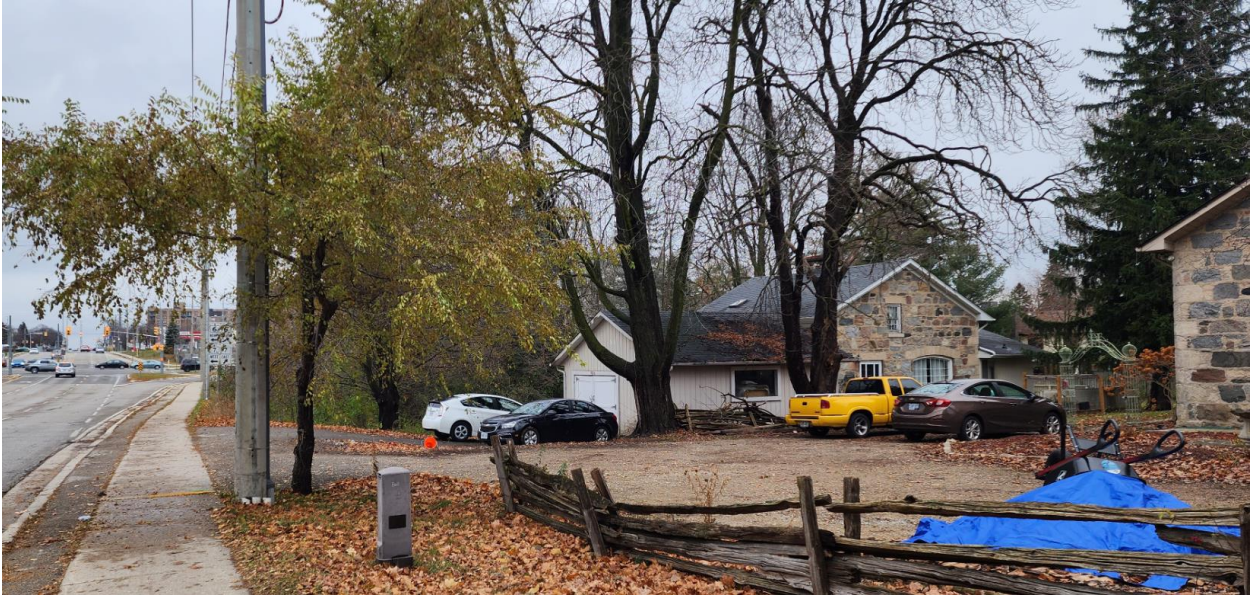
Figure 6 - View east along south side of Willow Road showing stone carriage house at 404 Willow Road beyond driveway. (Photo: S. Robinson)
