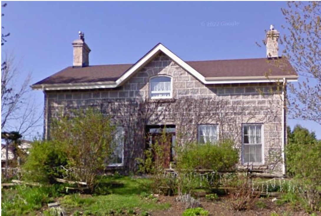
Figure 27: Photograph of 26 Kron Drive (Source: Google Streetview)
