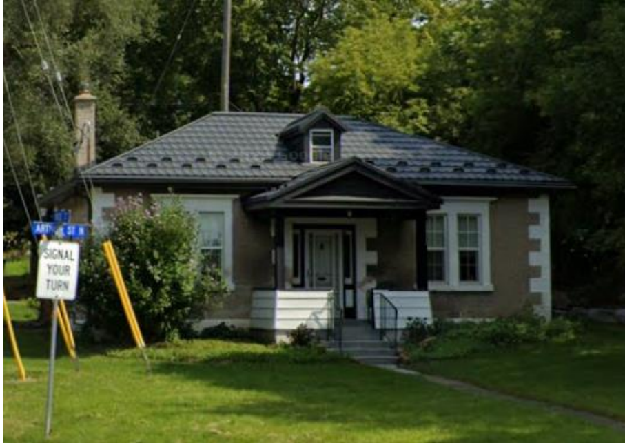
Figure 3: Photograph of 9 Arthur Street North (Source: Google Streetview)
