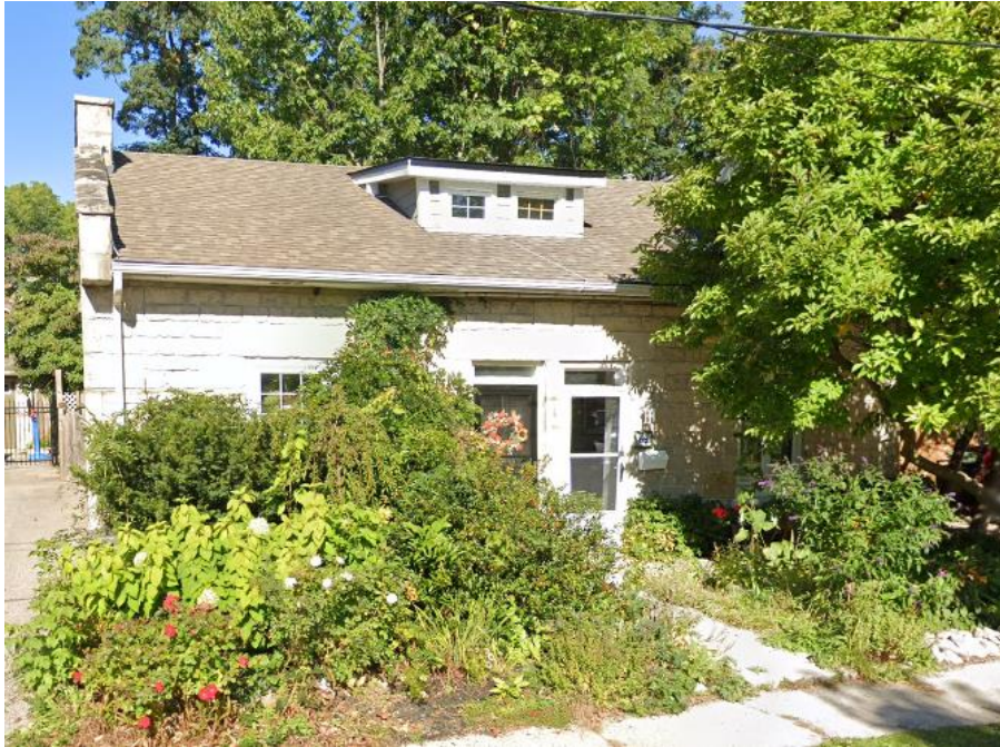
Figure 13: Photograph of 59/61 Essex Street (Source: Google Streetview)
