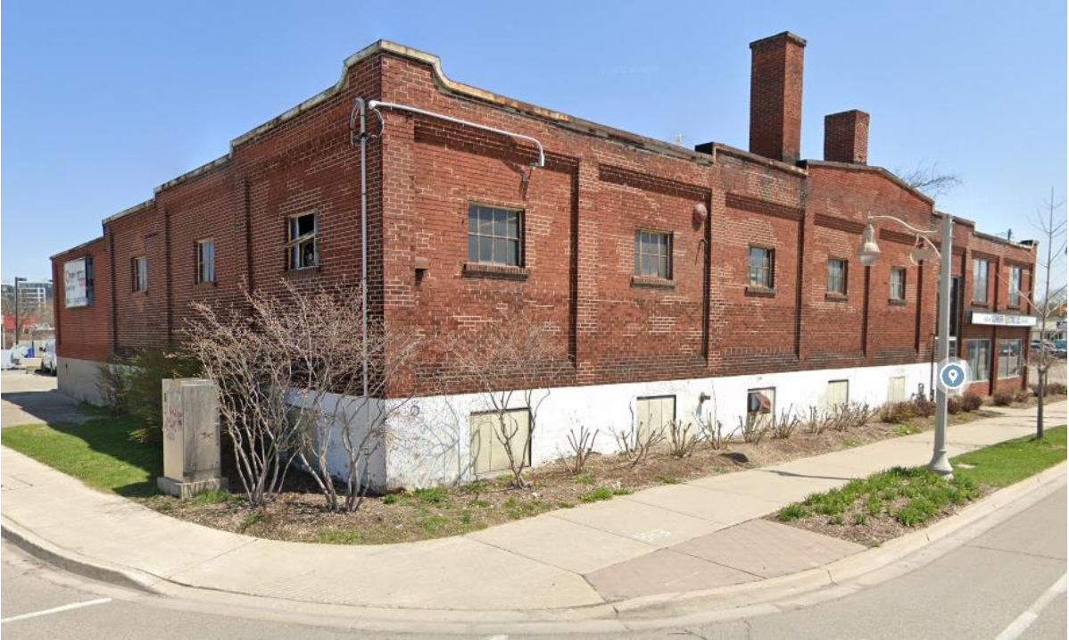
Figure 22: Photograph of 72 Gordon Street (Source: Google Streetview)
