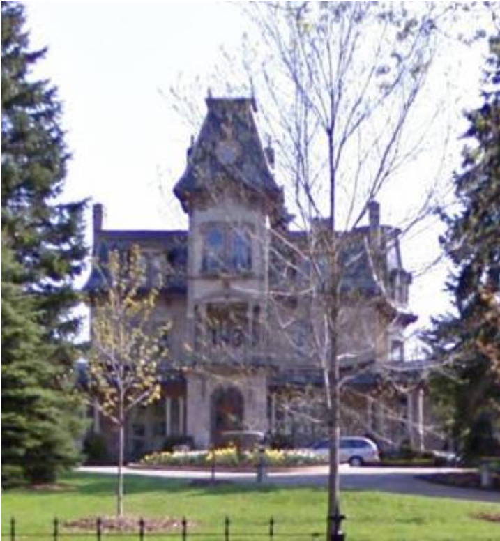
Figure 40: Photograph of 67 Queen Street (Source: Google Streetview)
