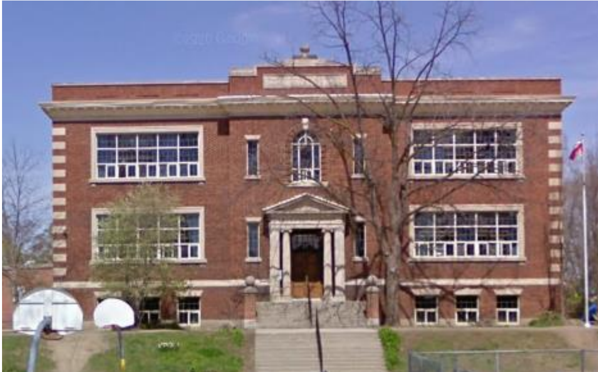
Figure 14: Photograph of Victory Public School (Source: Google Streetview)
