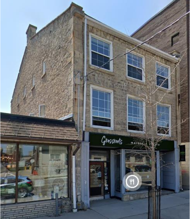
Figure 21: Photograph of 15 Gordon Street (Source: Google Streetview)
