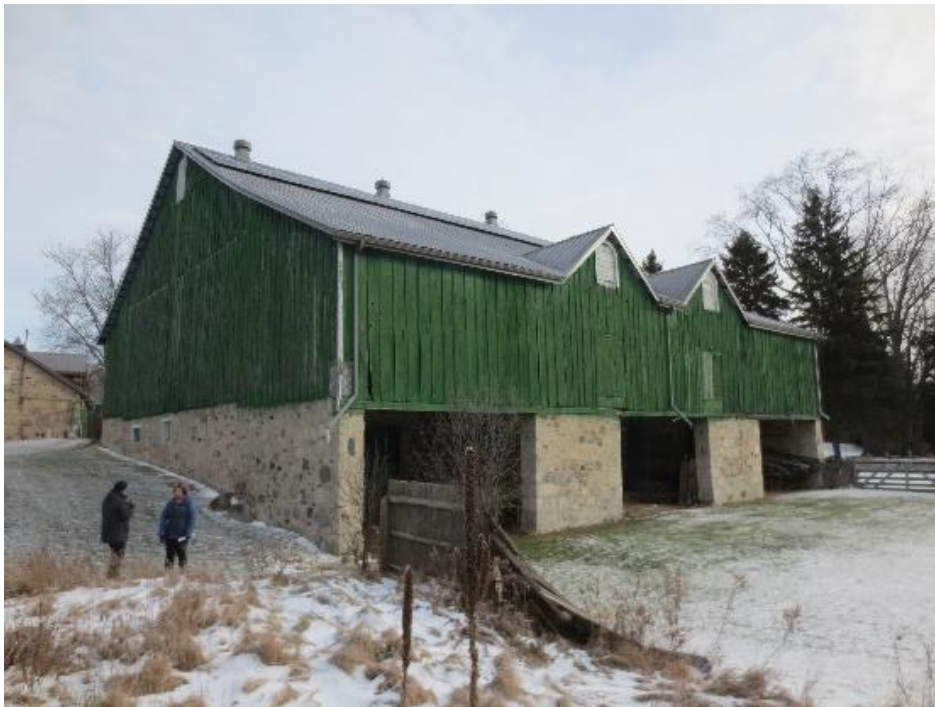
Figure 34: Photograph of bank barn at 35 Niska Road (Source: Heritage Planning Staff)
