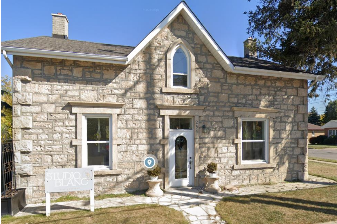
Figure 9: Photograph of 254 Edinburgh Rd S (Source: Google Streetview)
