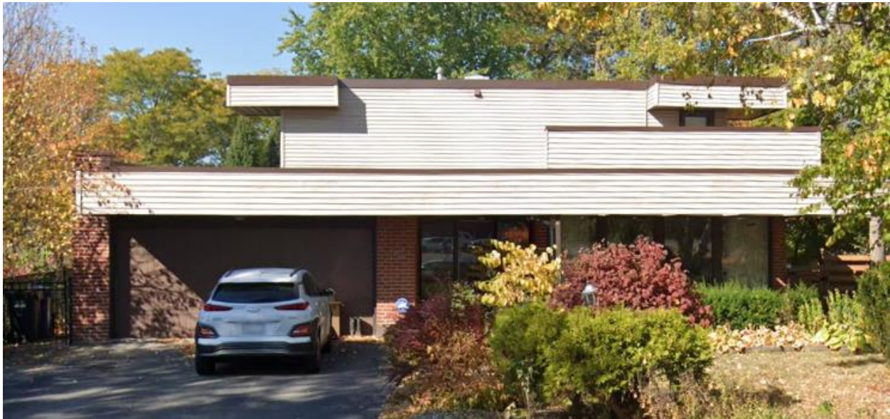
Figure 10: Photograph of 170 Emma Street (Source: Google Streetview)
