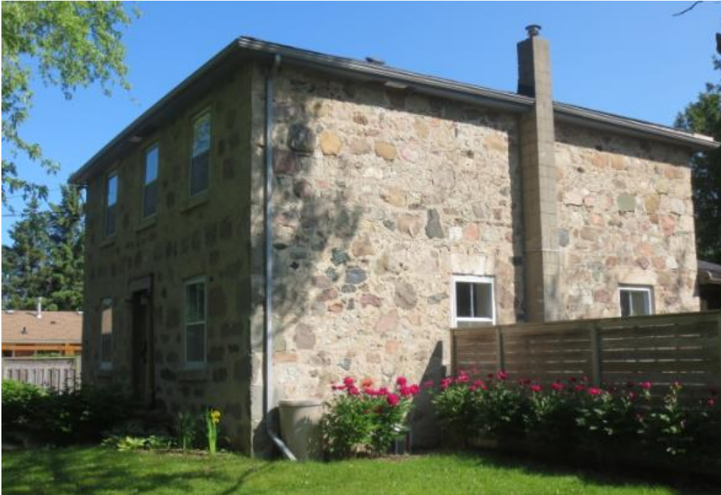
Figure 15: Photograph of 28 Ferndale Drive (Source: Heritage Planning Staff)
