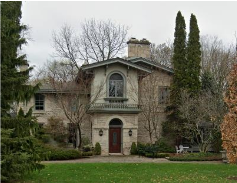
Figure 45: Photograph of 19 Woodycrest Drive (Source: Google Streetview)
