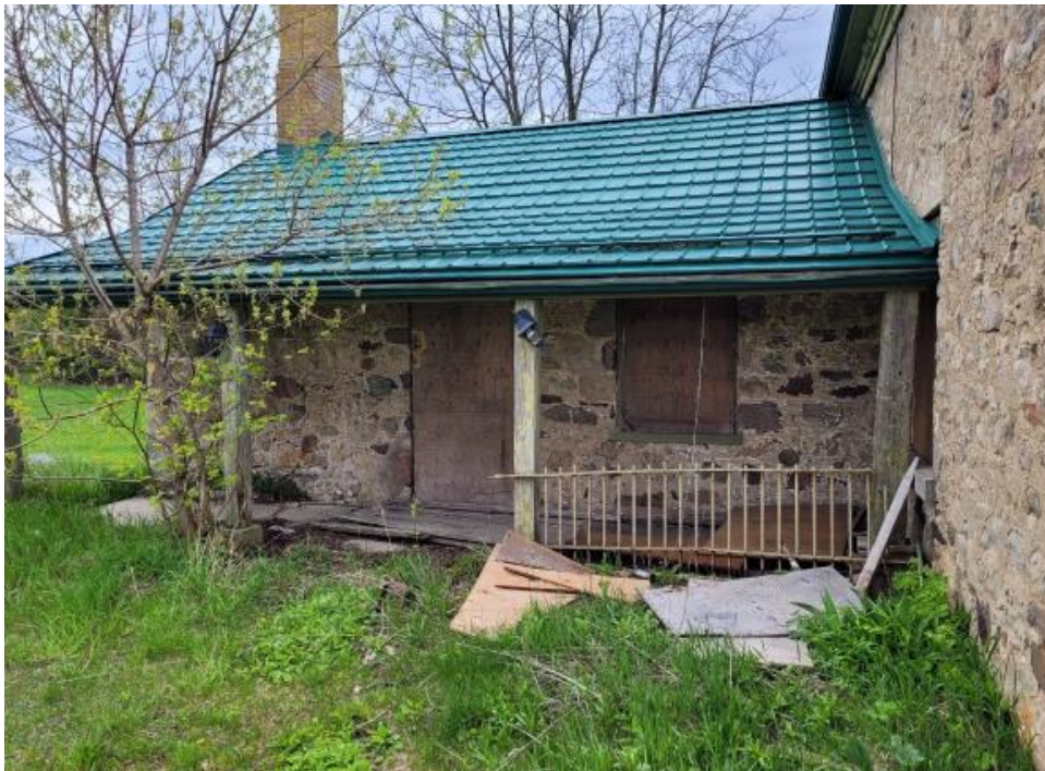
Figure 2: East elevation of the summer kitchen (photo: MHBC)
