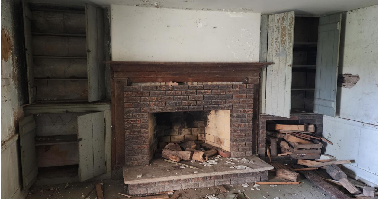
Figure 5: South interior wall of summer kitchen (photo: Heritage staff, 2023)
