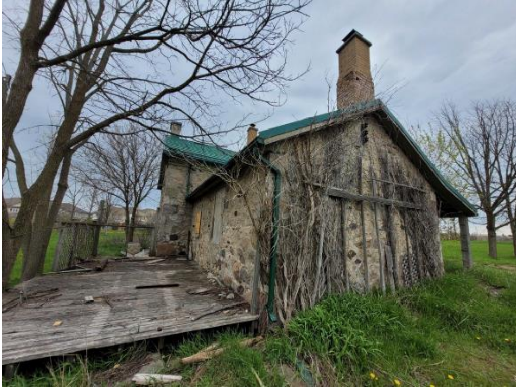
Figure 3: Rear (South) elevation of the summer kitchen (photo: MHBC)
