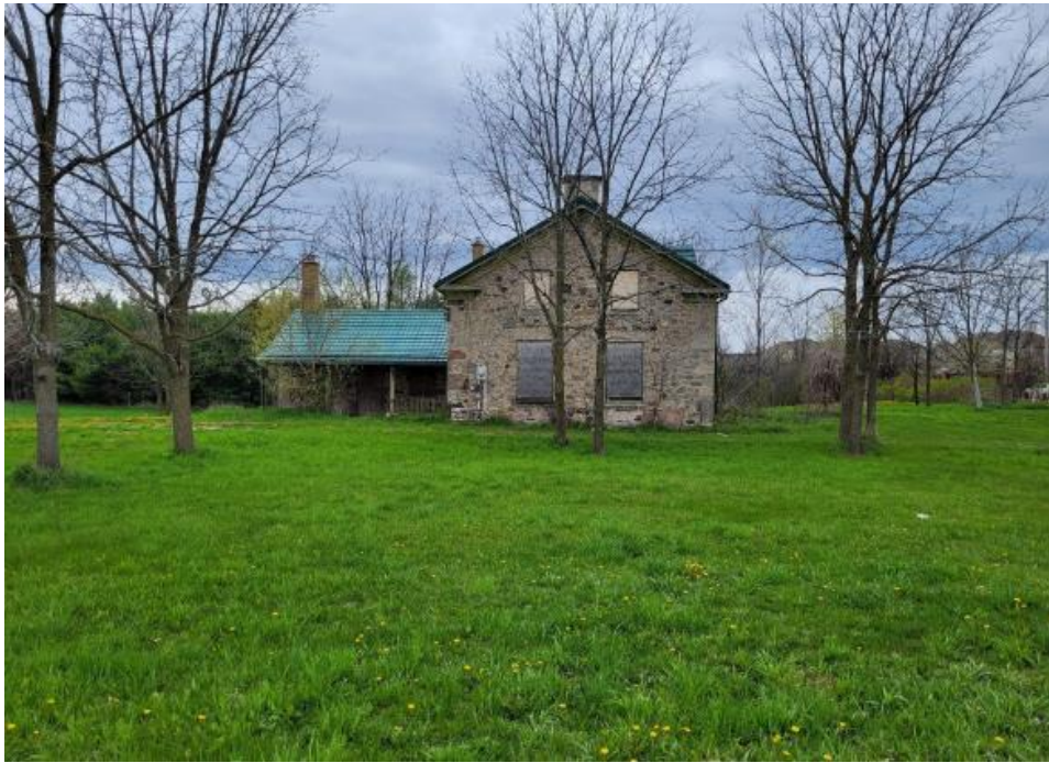
Figure 1: East elevation of the summer kitchen and main house (photo: MHBC)
