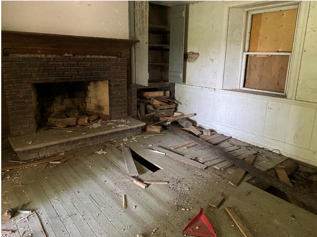
Figure 6: Southwest corner of summer kitchen interior (photo: Heritage staff, 2023)
